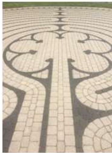
The individuals that contacted us estimated that this work could be completed at a cost between \$10,000 and \$20,000. Ongoing maintenance would consist of cleaning and sealing the pavers every three to five years; re-staining should not be needed.
