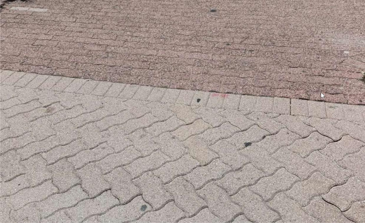
Brick manufacturers now add chemicals to the upper one quarter of an inch of the pavers to provide a better finish that holds its color better and cleans up better when power washed. Below is the new standard paver that is used in downtown Naperville which is manufactured by Unilock.
