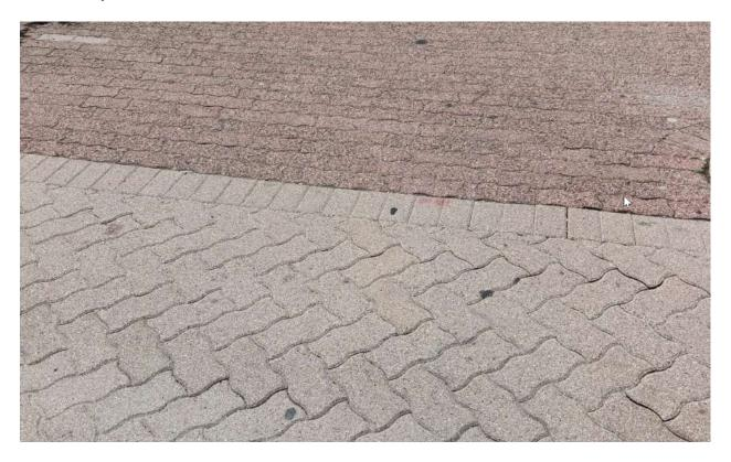
Brick manufacturers now add chemicals to the upper one quarter of an inch of the pavers to provide a better finish that holds its color better and cleans up better when power washed. Below is the new standard paver that is used in downtown Naperville which is manufactured by Unilock.
