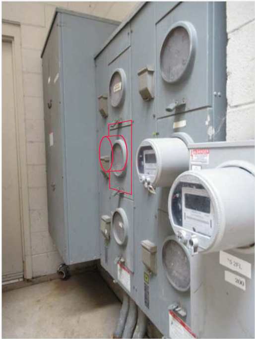
PROPOSED ELECTRICAL SERVICE METER TO BE INSTALLED AT EXISTING MULTI-GANG METER BANK NEAR EXISTING TRANSFORMER
