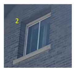
Remove and replace window unit with double hung clear glass.
