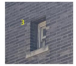
Remove and replace window unit with double hung clear glass.
