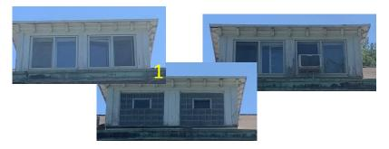
3 Roof Dormers: Remove and replace window units with like style units with clear glass.
