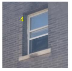
Remove and replace window unit with double hung clear glass.
