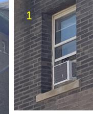
Remove and replace window unit with double hung clear glass.
