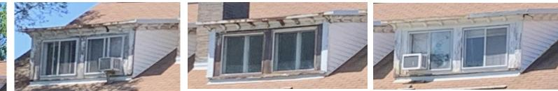
3 Rear Roof Dormers: Remove and replace window units with like style units with clear glass.
