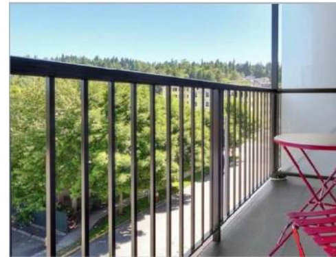
METAL BALCONY RAILING
