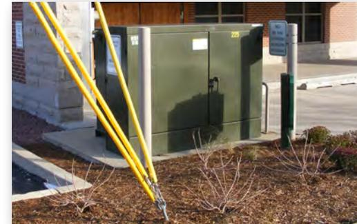
**Image 25:** The preferred location for a transformer is on a rear facade where adequate service access is provided.
