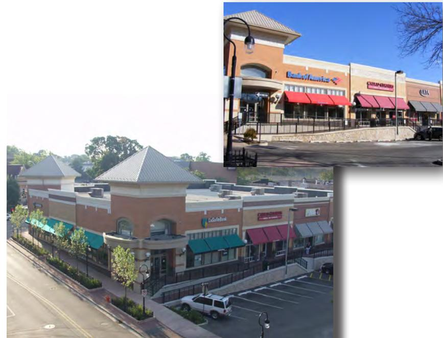
**Image 10:** Parapets are used to screen rooftop units so that they are not visible from the ground level
