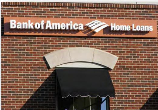
**Image 28:** Individual letters are applied to a panel to minimize damage to underlying masonry. Colors are complementary to the building.
