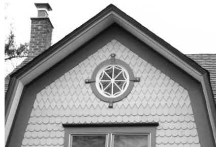
Photo D.16 - Shingle style residence with decorative glass - 119 N. Brainard Street
