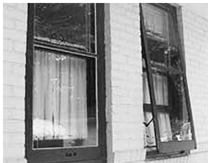
Photo D.12 - 1920's residence with original wood storms, Oak Park, Illinois
