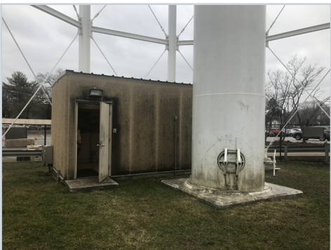
Efficient Demolition: Keeping Radio Equipment in Service During Tank Construction
