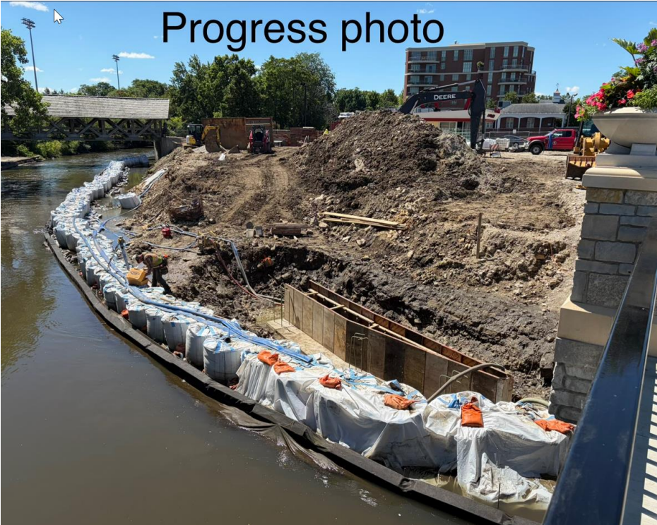
Cofferdam and low flow walk from the Washington Street Bridge
