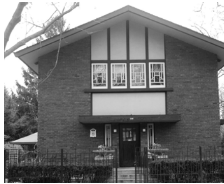
Photo C.17 - Prairie style residence with brick siding, stucco accents and wood trim - 144 S. Sleight Street
