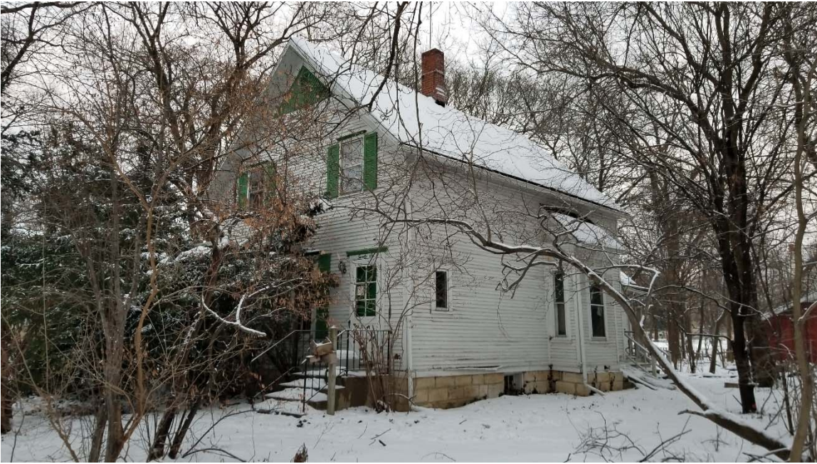
Image 1 – Existing house from southwest corner
