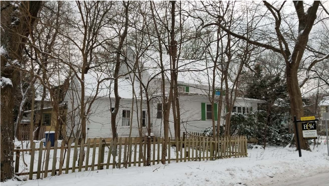
Image 3 – East addition from northeast corner
