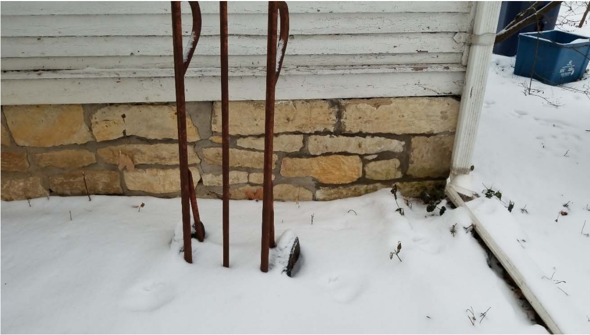
Image 19 – Stone foundation with signs of patching
