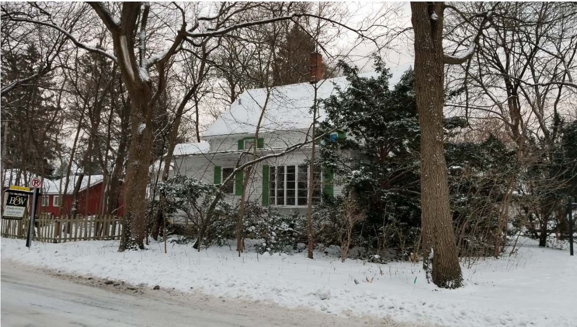
Image 2 – North addition from northwest corner
