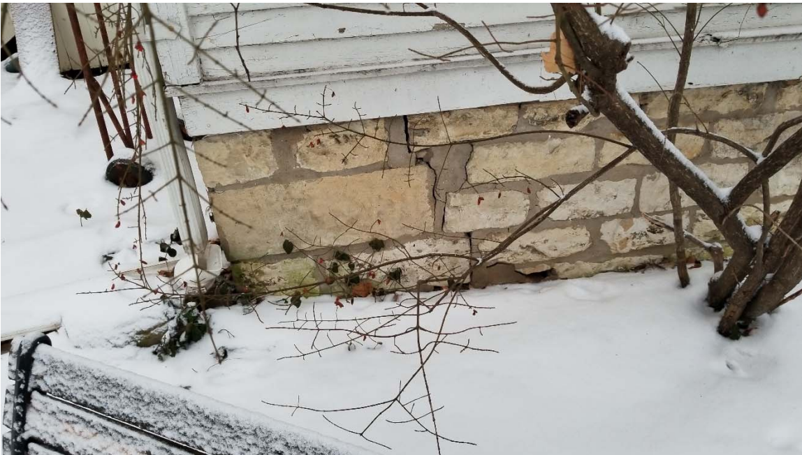
Image 20 - Stone foundation with signs of patching
