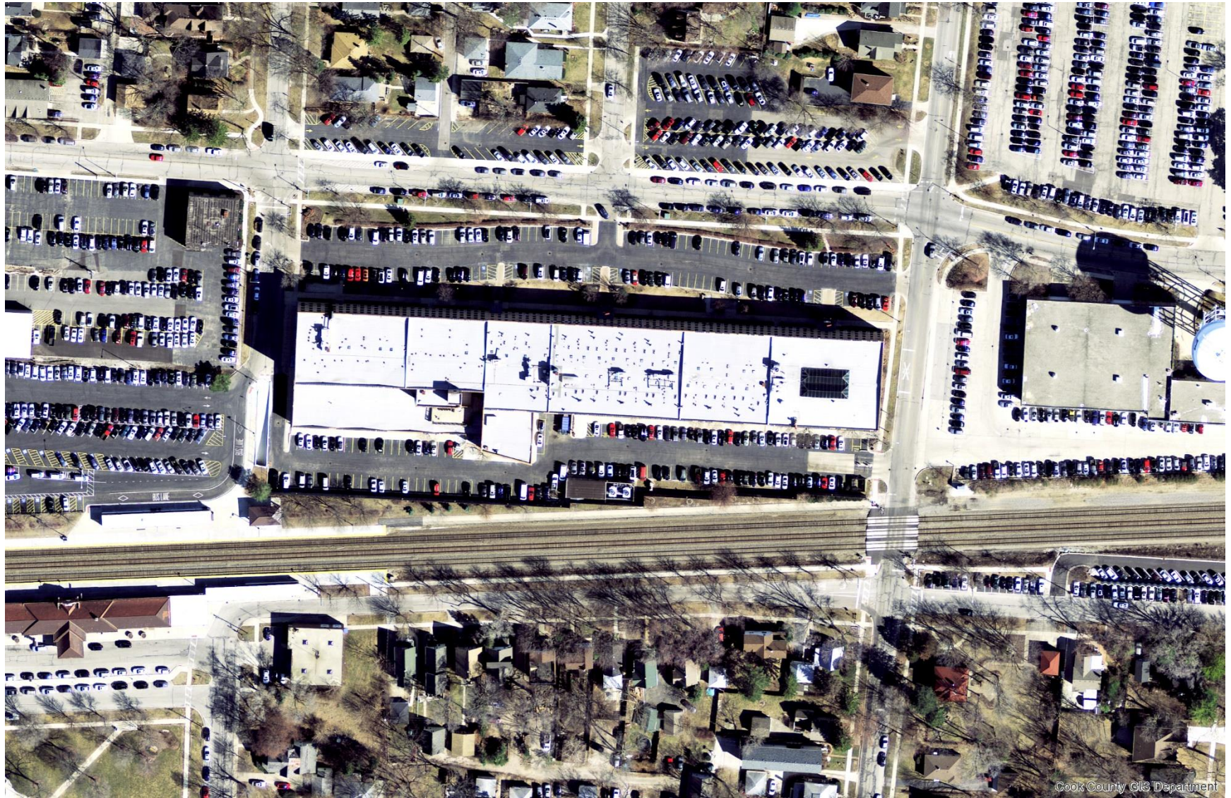
Figure 3 AERIAL PHOTOGRAPH – COOK COUNTY GIS DEPARTMENT – 2013
