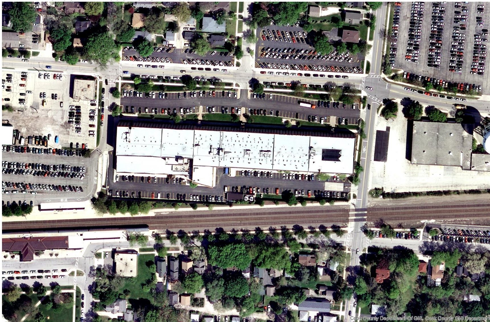
Figure 1 AERIAL PHOTOGRAPH – COOK COUNTY GIS DEPARTMENT – 2009
