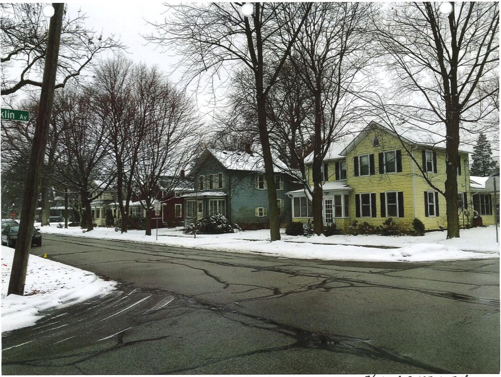
S/W CORNER VIEW
