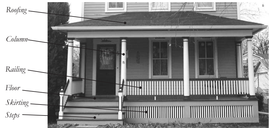
Photo D.34 - Porch Components - 5 N. Sleight Street
