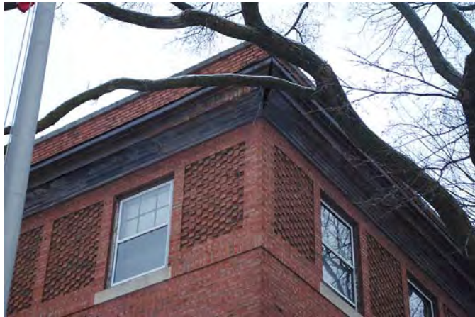
Brick diaper pattern at third story
