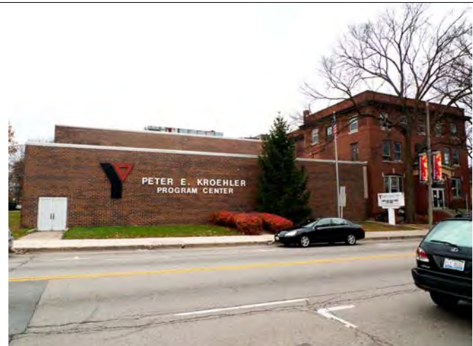
North side addition
