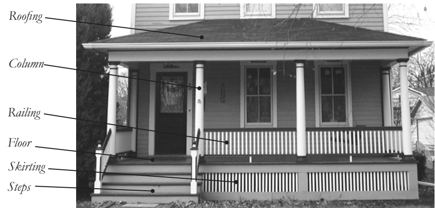
Photo D.34 - Porch Components - 5 N. Sleight Street
