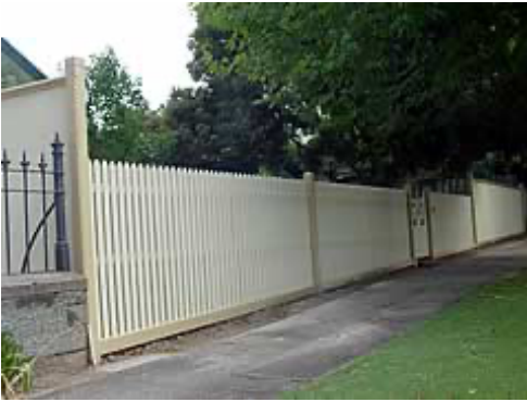
A sloping plinth throughout both styles of fence yet maintaining a window sill line on the home behind.
