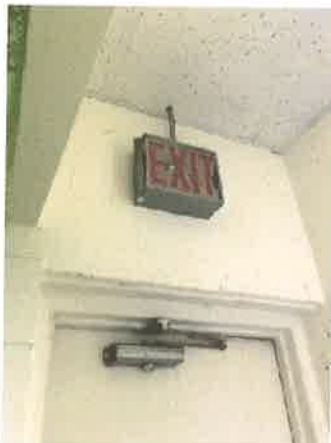
Exit Signage Replacement 1
