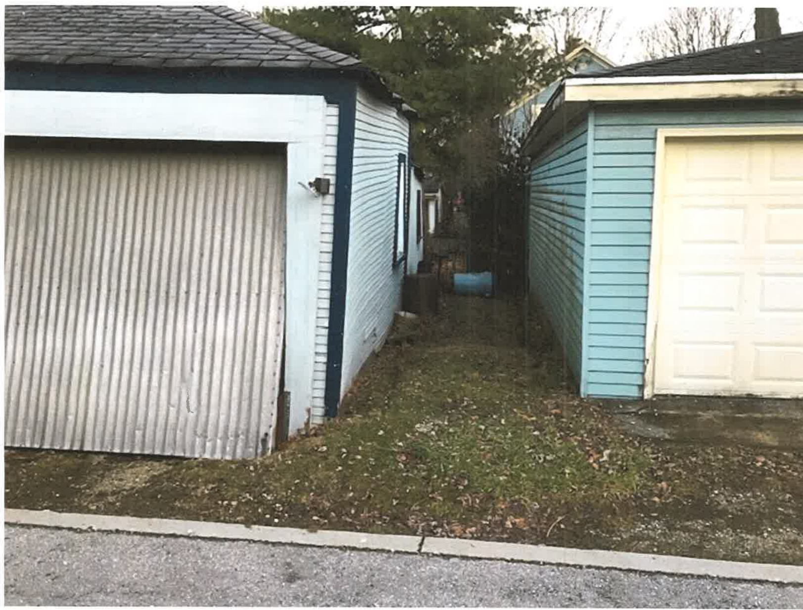
SOUTH FACING SIDE OF GARAGE
