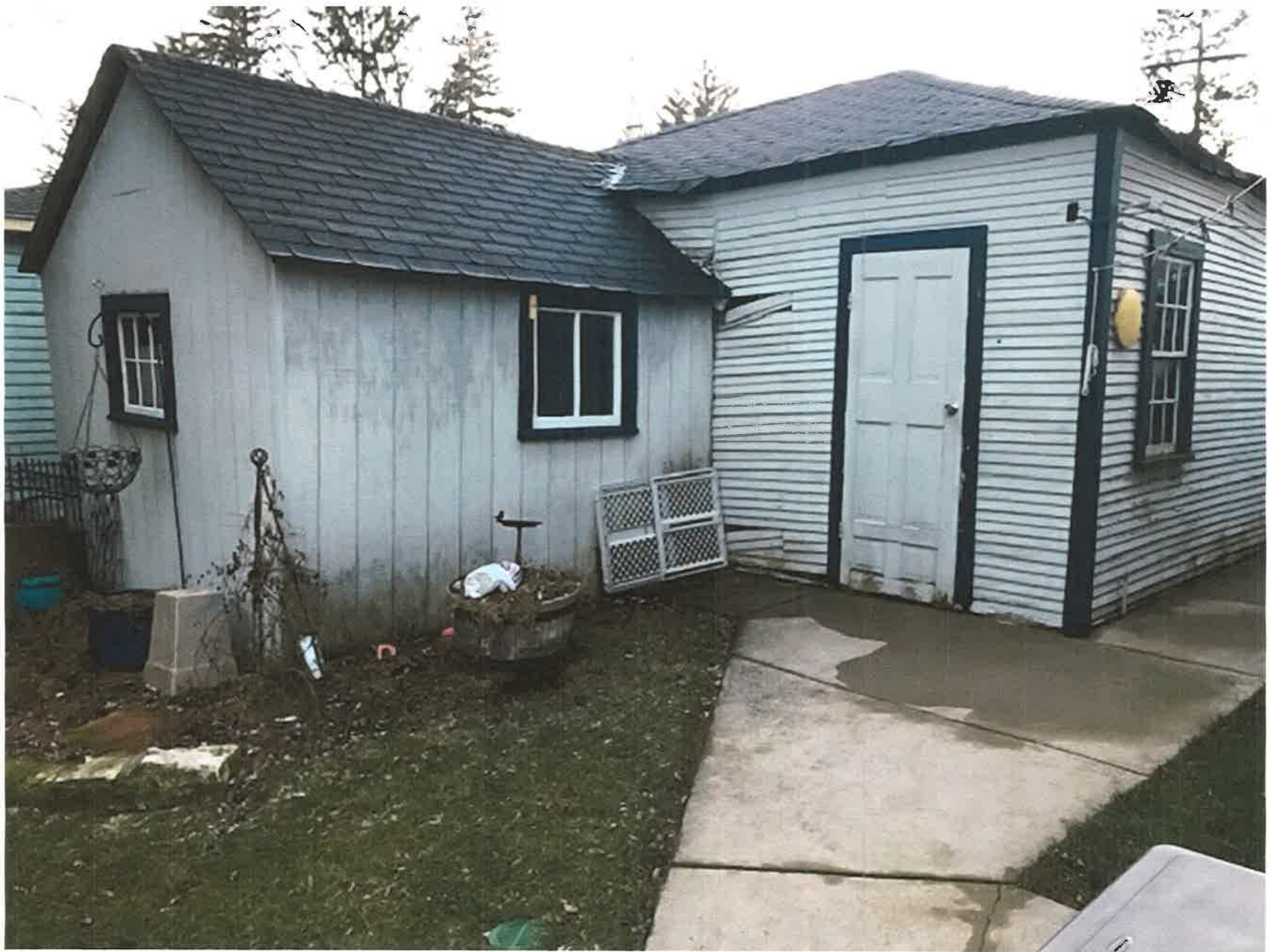
SERVICE DOOR ON EAST SIDE OF GARAGE (CLOSE TO NORTH SIDE)
