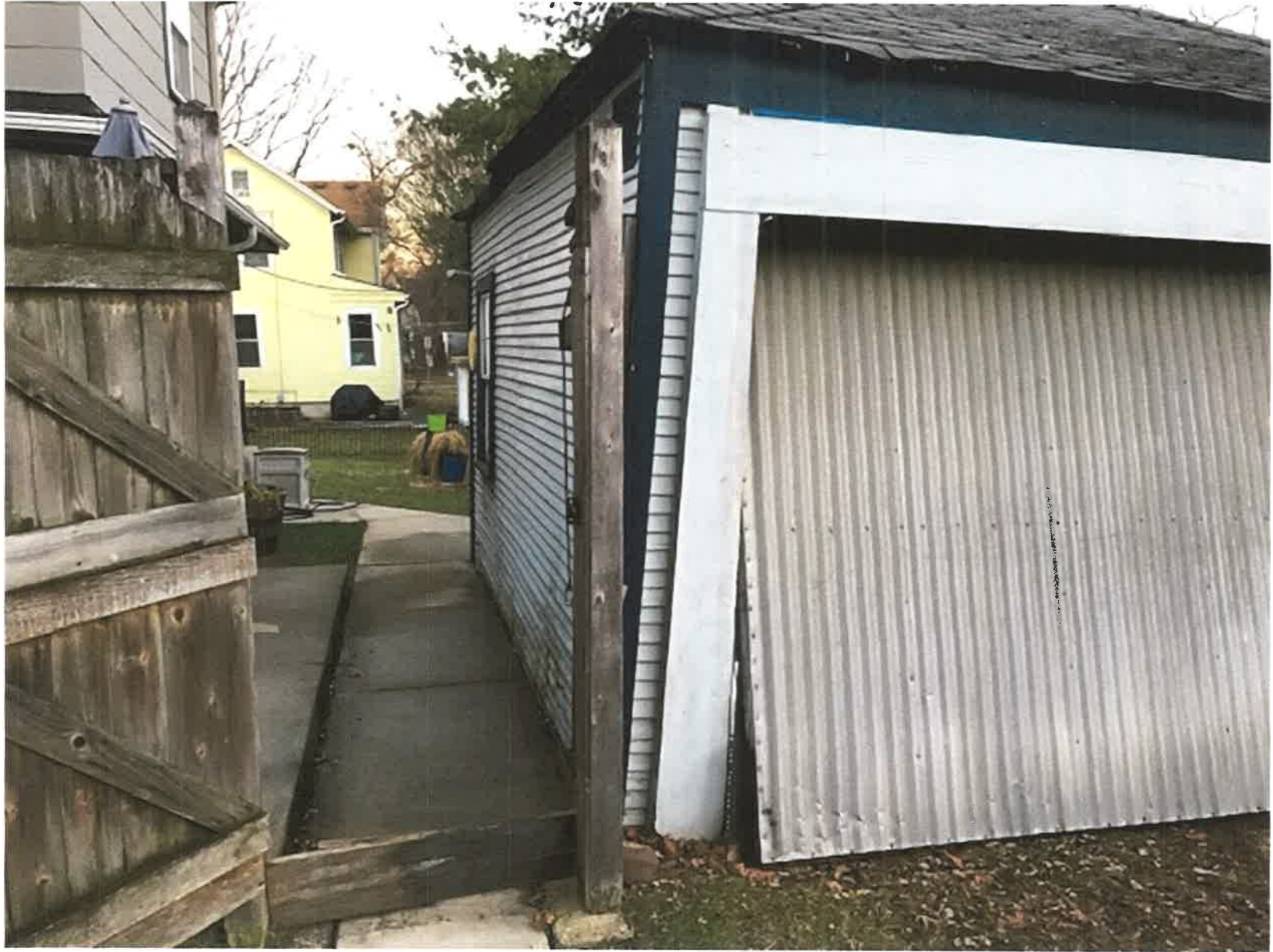
NORTH FACING SIDE OF GARAGE
