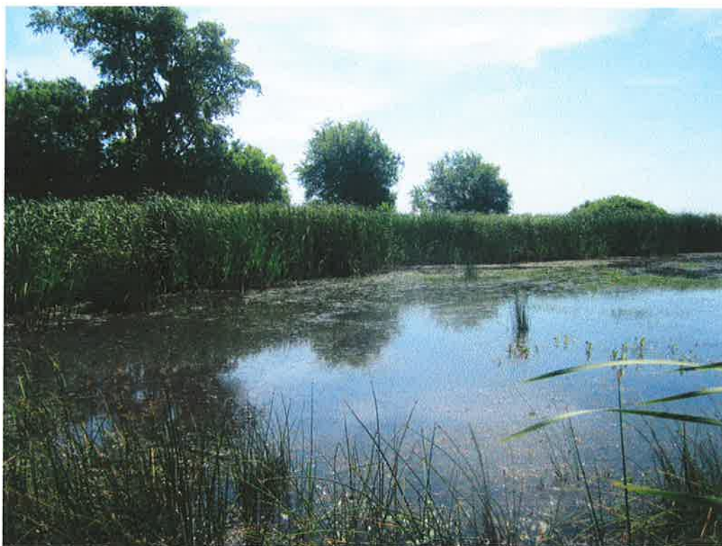
Figure 3—Facing south at corner of detention basin. Photo taken 6/08/12.
