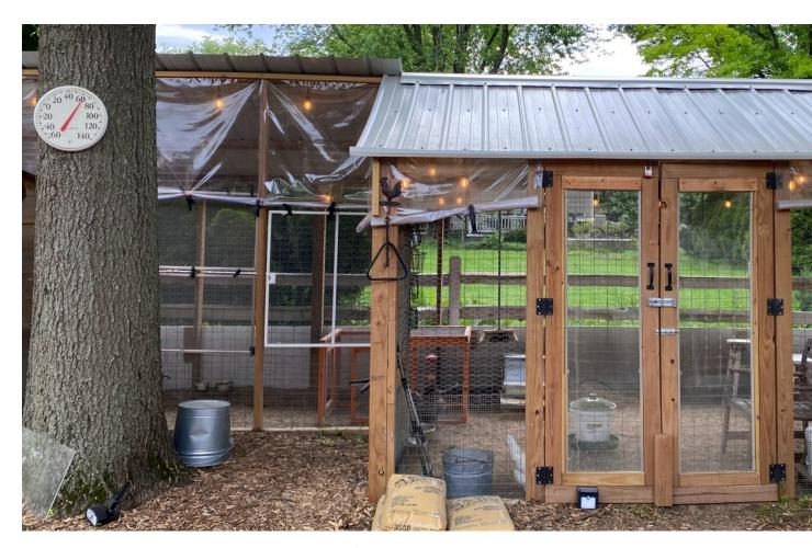
Run 1 is completely enclosed with a combination of standard chicken wire and heavy gauge rectangular wiring similar to screening used in the coops.
