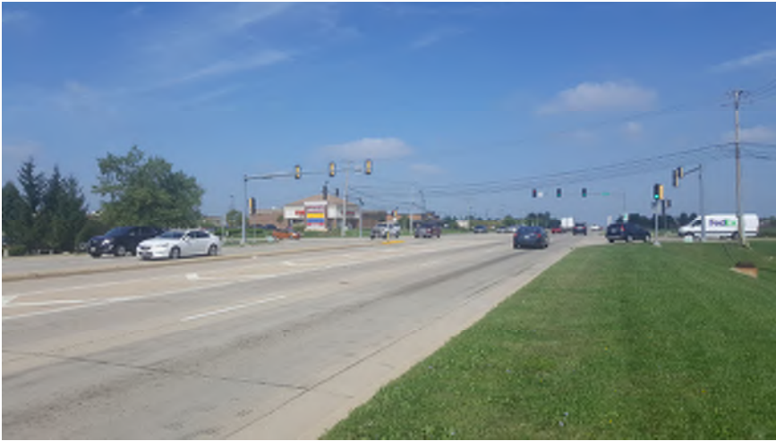
Northbound IL 59 (119 th St intersection)
