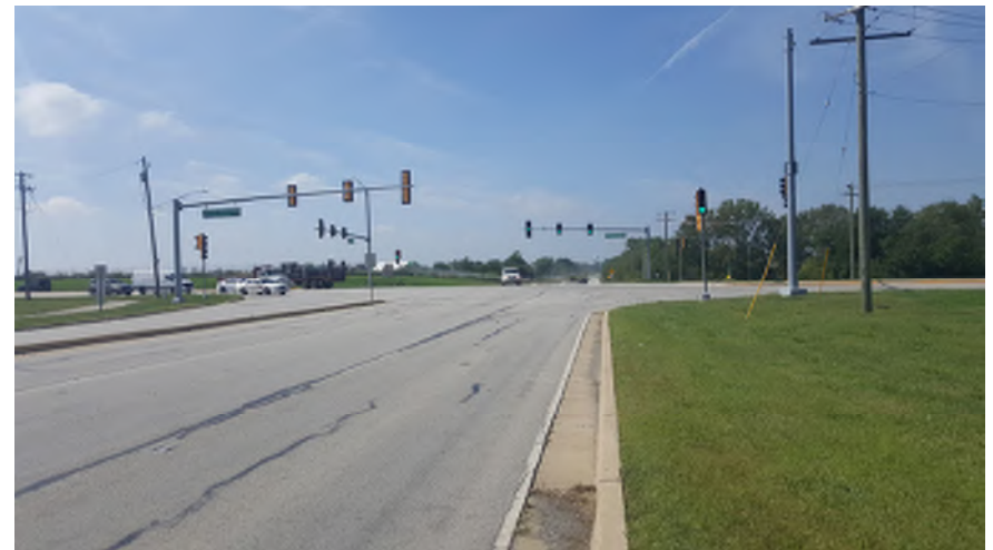
Westbound 119 th St (Plainfield-Naperville Rd intersection)
