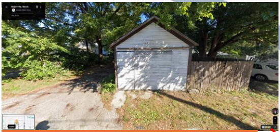
516 Current garage structure
