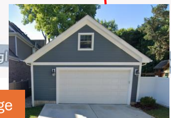
2 story detached garage
