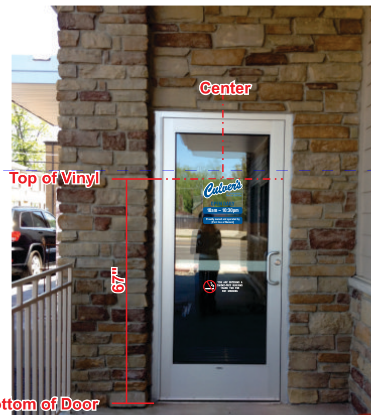
Typical Installation Example - Drive-Up Entrance
