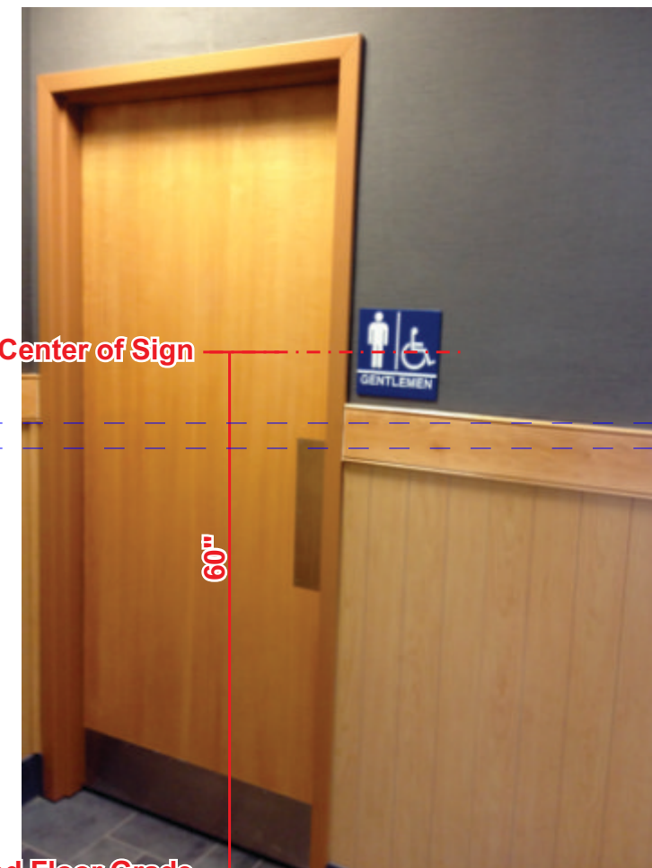
Finished Floor Grade Typical Installation Example -
