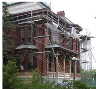
MARTIN MITCHELL MANSION RESTORATION
