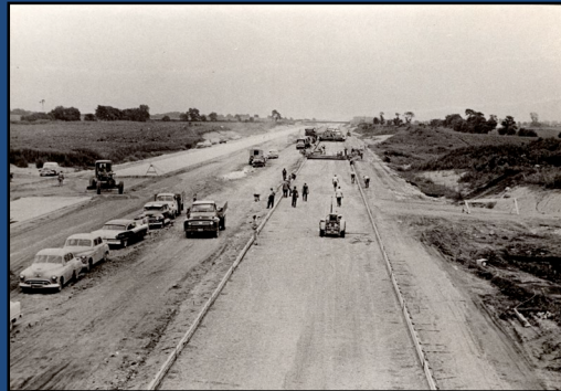
Construction of the I-88 Tollway Photo credit: Mary Lou Wehrli
