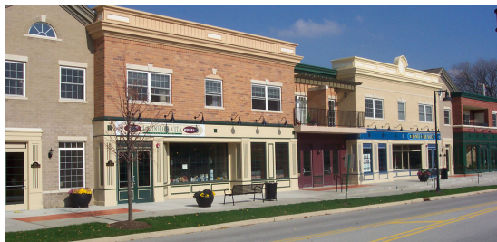
Mix Of Uses, Including Retail Stores, Restaurants & Offices
