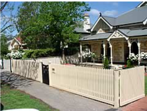
Clean lines and simple forms compliment the house best.
