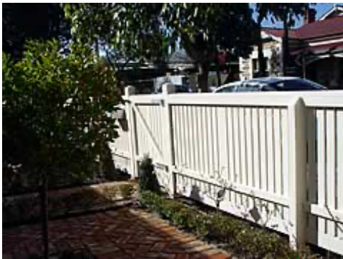
Structural posts are hidden from the street view.
