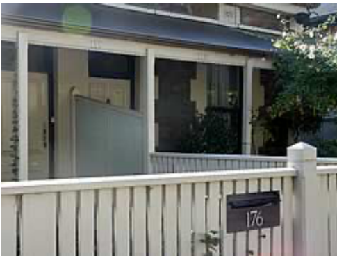
Between hose wall & verandah post a 2-sided galvanised ripple screen.
