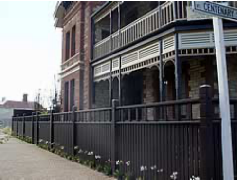
The circular motiff & multiple collars reflect the decorative verandah posts.
