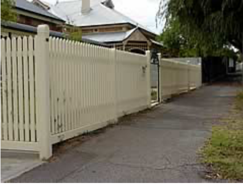
Almost a metre fall in this site but the fence is still square to the house behind.
