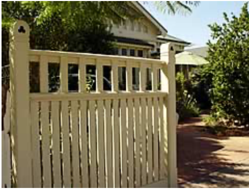
Split level fences allow for pickets or mini-flute in the base section.
