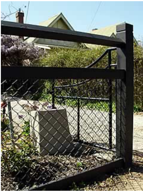
The original gate reinstated with a mortice diamond rail used above chainwire for a hedge to grow.
