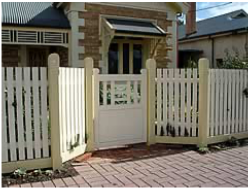
Flat top pickets are a genuine detail coupled with a gate that mimics the fretwork.
