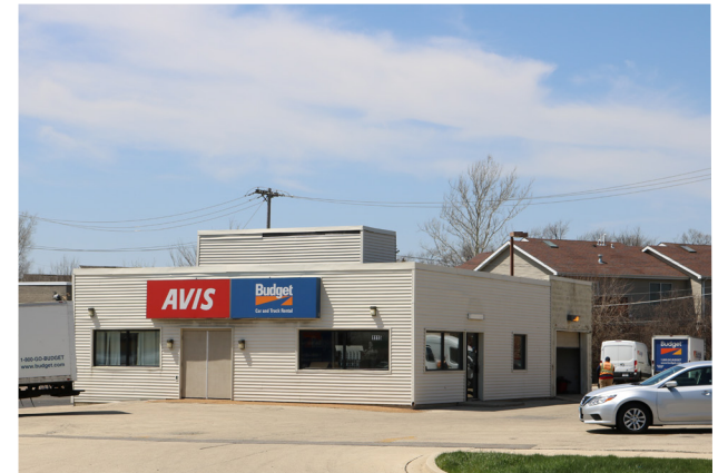
1115 E Ogden Ave Avis/Budget Rental Facade sign
