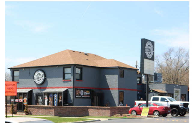
909 E Ogden Ave Crosstown Pub Pole Sign
