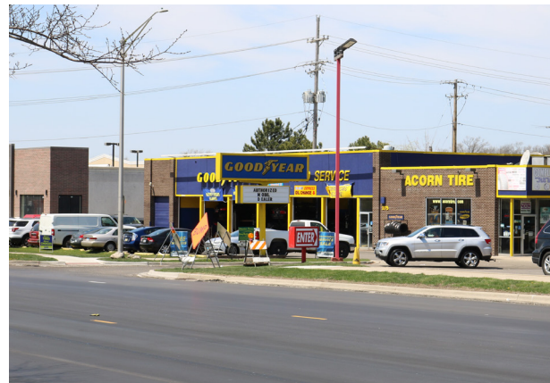
275 E Ogden Ave Good Year Tire Pole Sign
