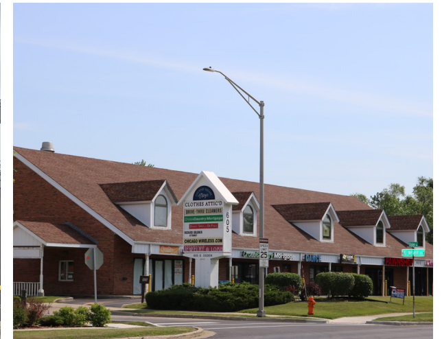
605 E Ogden Ave Country Square Plaza Pole Sign
