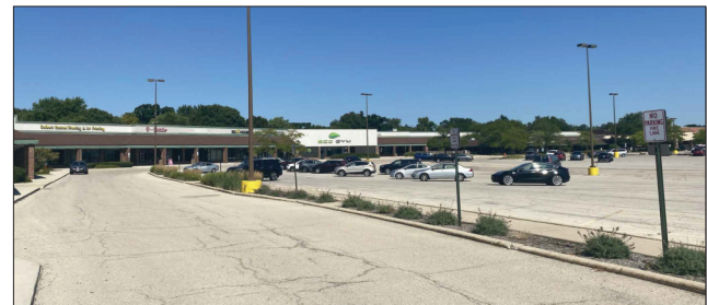
B EXISTING PHOTOGRAPH SCALE: NIS
