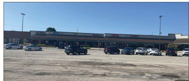
C EXISTING PHOTOGRAPH SCALE: NIS
