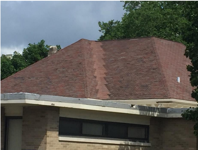
Figure 34. South roofing face.
