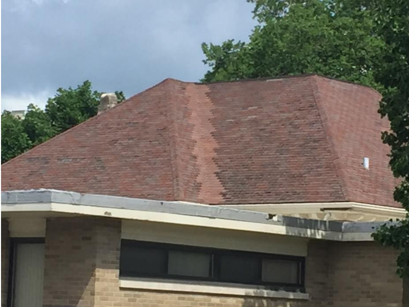
Figure 42. Another location of previous valley repair.
