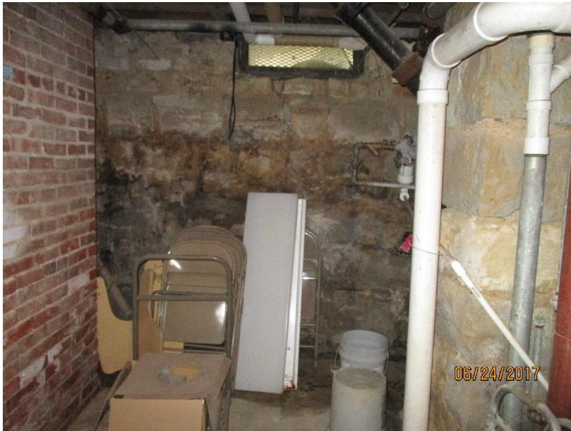
Figure 26. Partial view of west end of north foundation wall.
