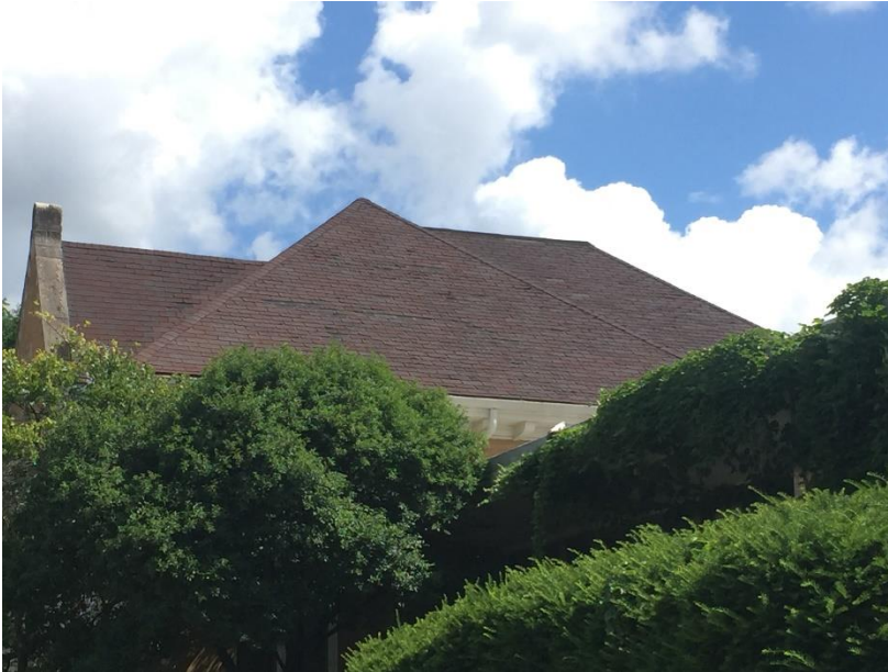
Figure 33. South roofing face.
