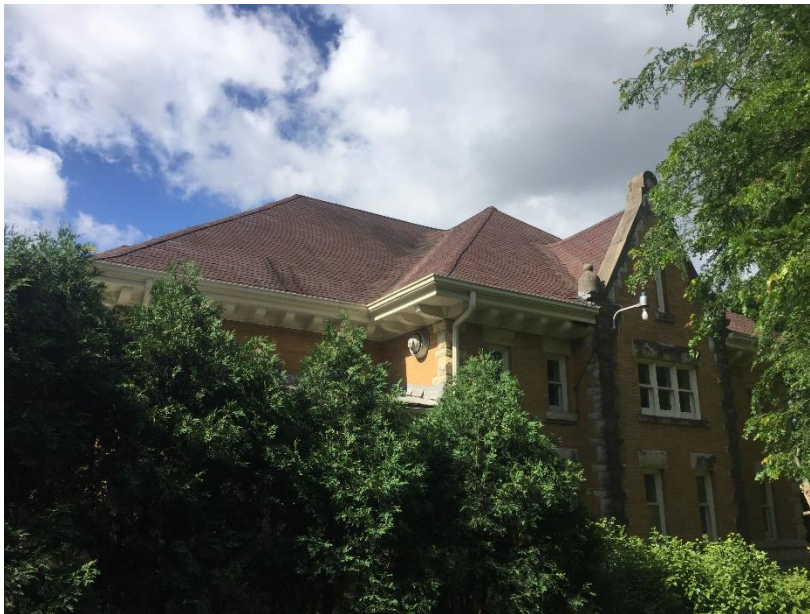
Figure 36. North roofing face.
