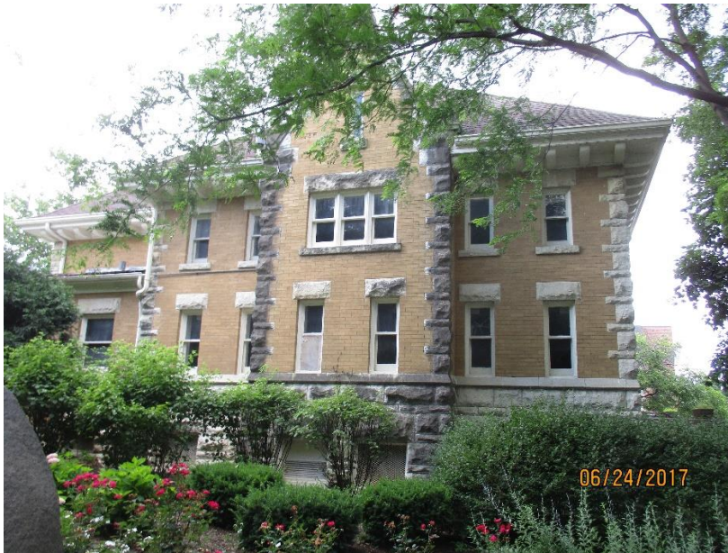
Figure 4. Overall view of north facade
