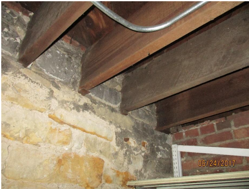
Figure 28. No evidence of decay on wood framing.
