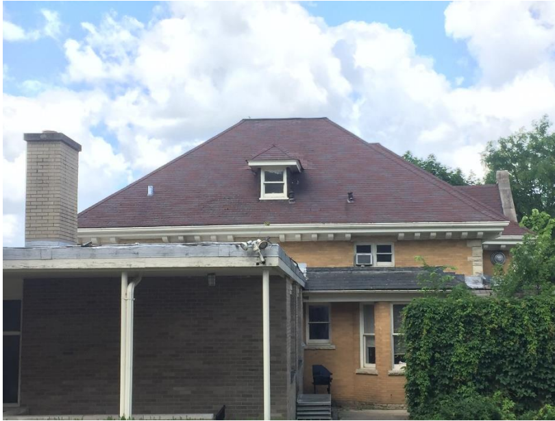
Figure 35. East roofing face.
