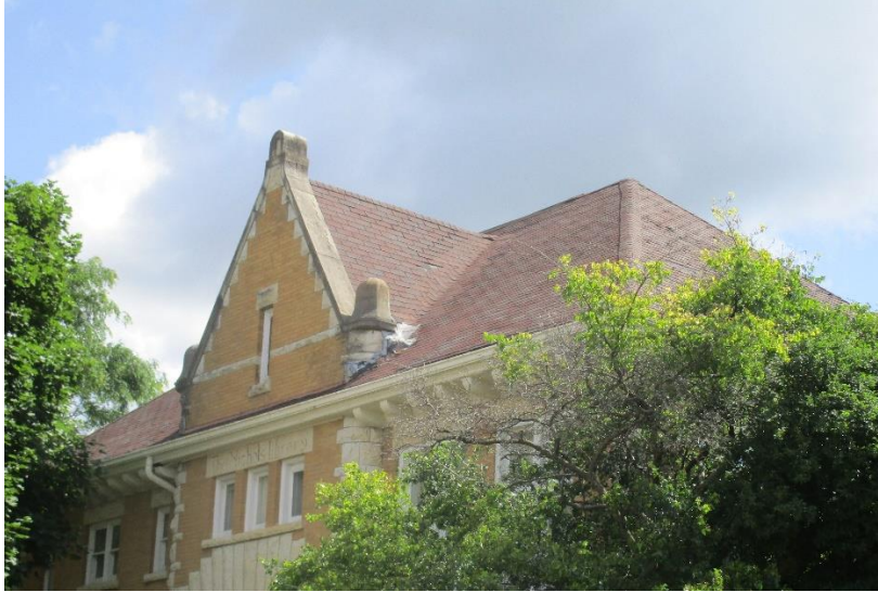
Figure 37. West roofing face (from southwest corner).
