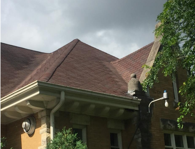
Figure 41. Location of previous valley repair.
