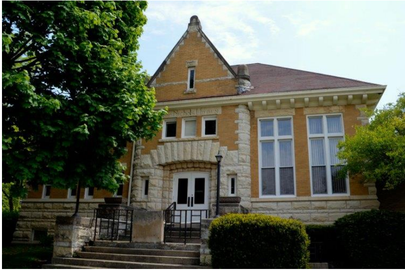
Figure 1. Over all view of the west facade of Old Nichols Library.
