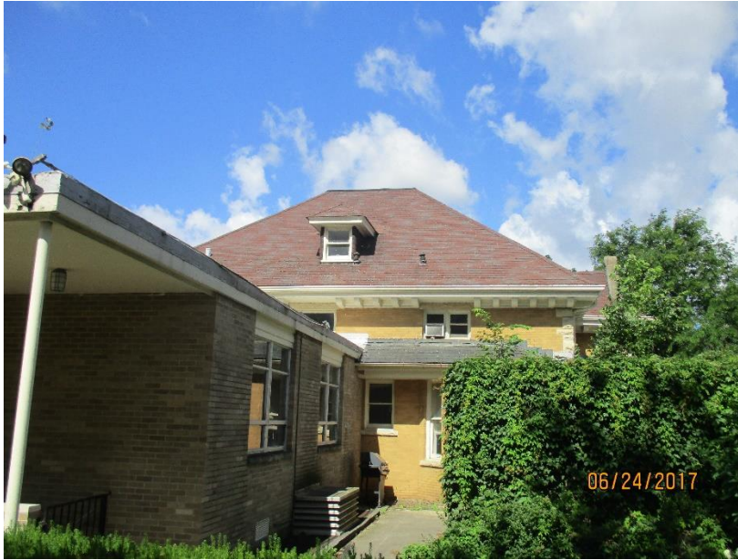
Figure 3. Partial view of east facade.
