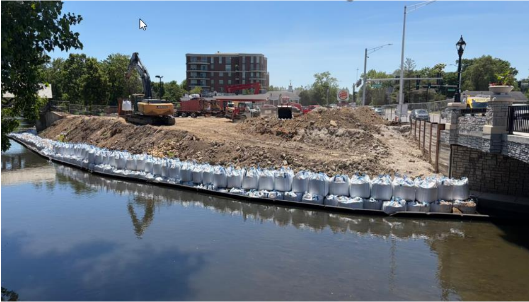
Cofferdam Installation
