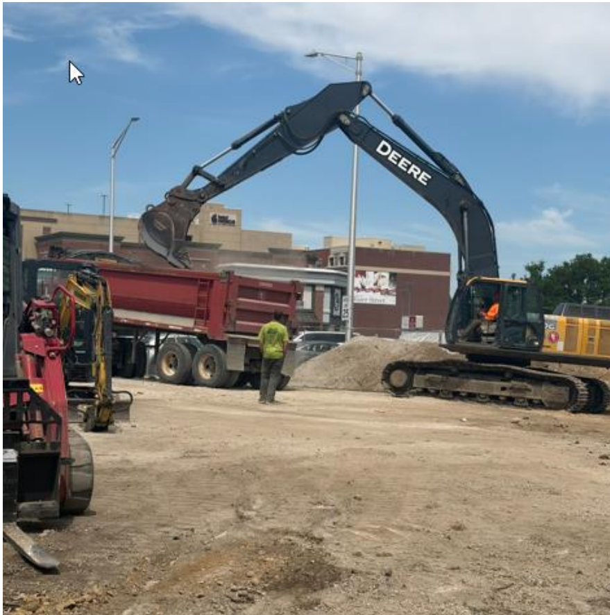
Initial Soil Excavation
