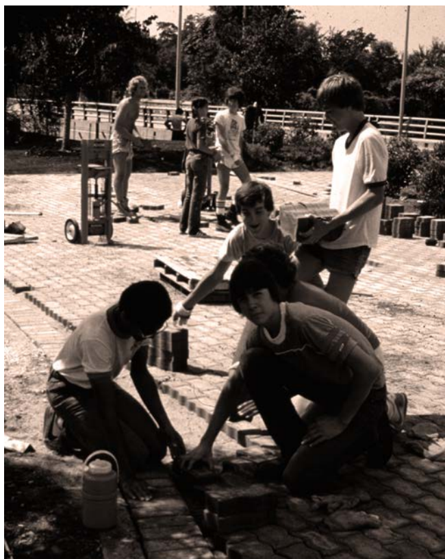
Volunteers Lay Bricks - 1981
