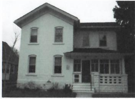
Photo C.16 - I-Form vernacular style residence - 214 N. Ellsworth Street
