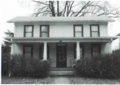
Photo C.15 - I-Form vernacular style residence - 154 Center Street
