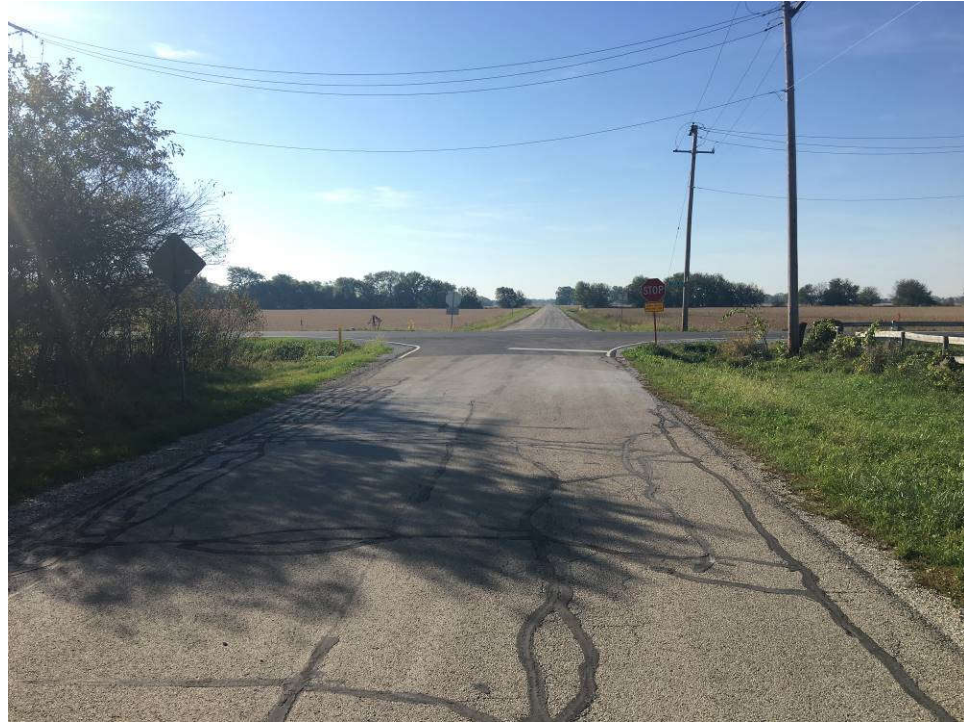
Looking south along Book Rd at 119 th St
