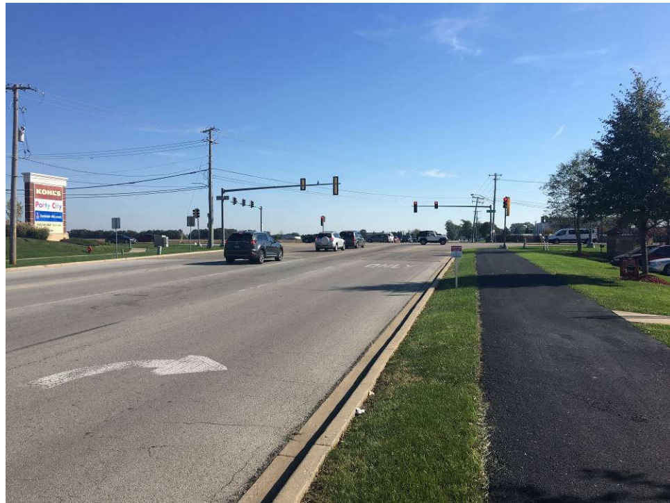
Looking east along 119 th St at IL 59
