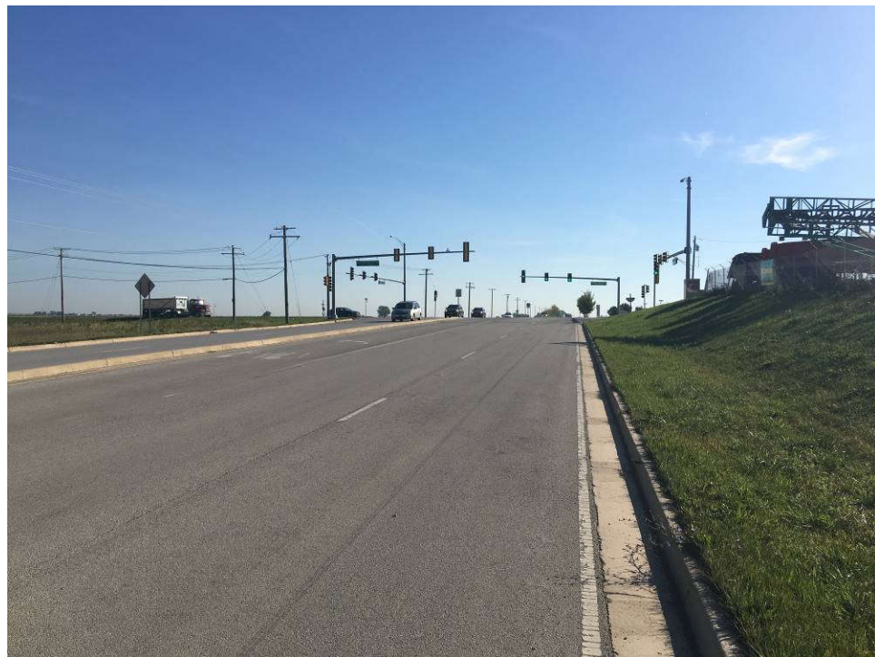
Looking east along 119 th St at Plainfield-Naperville Rd
