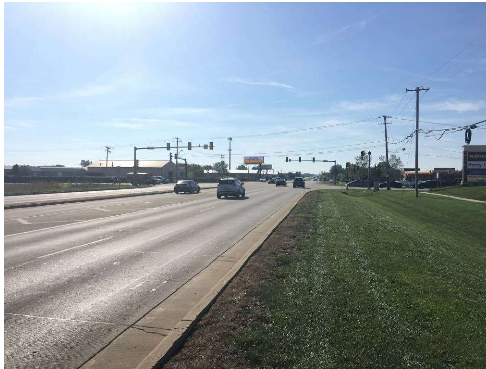
Looking south along IL 59 at 119 th St
