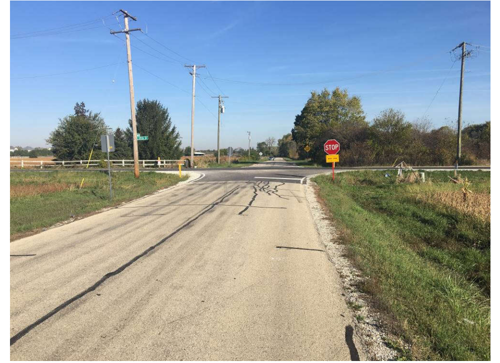
Looking north along Book Rd at 119 th St
