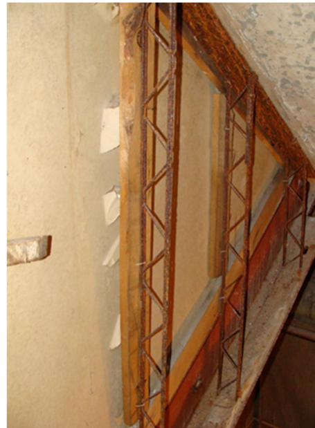
Photo #1 – Open web wall studs in 140
