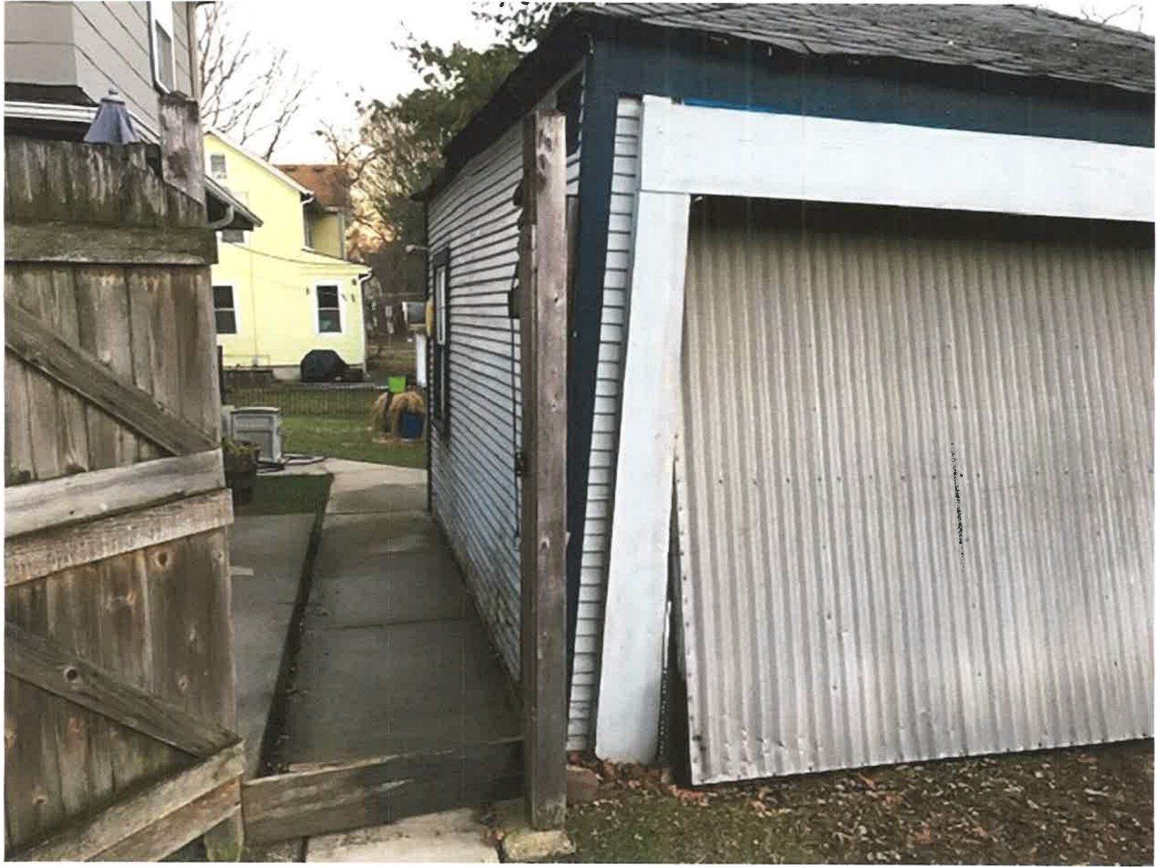
NORTH FACING SIDE OF GARAGE
