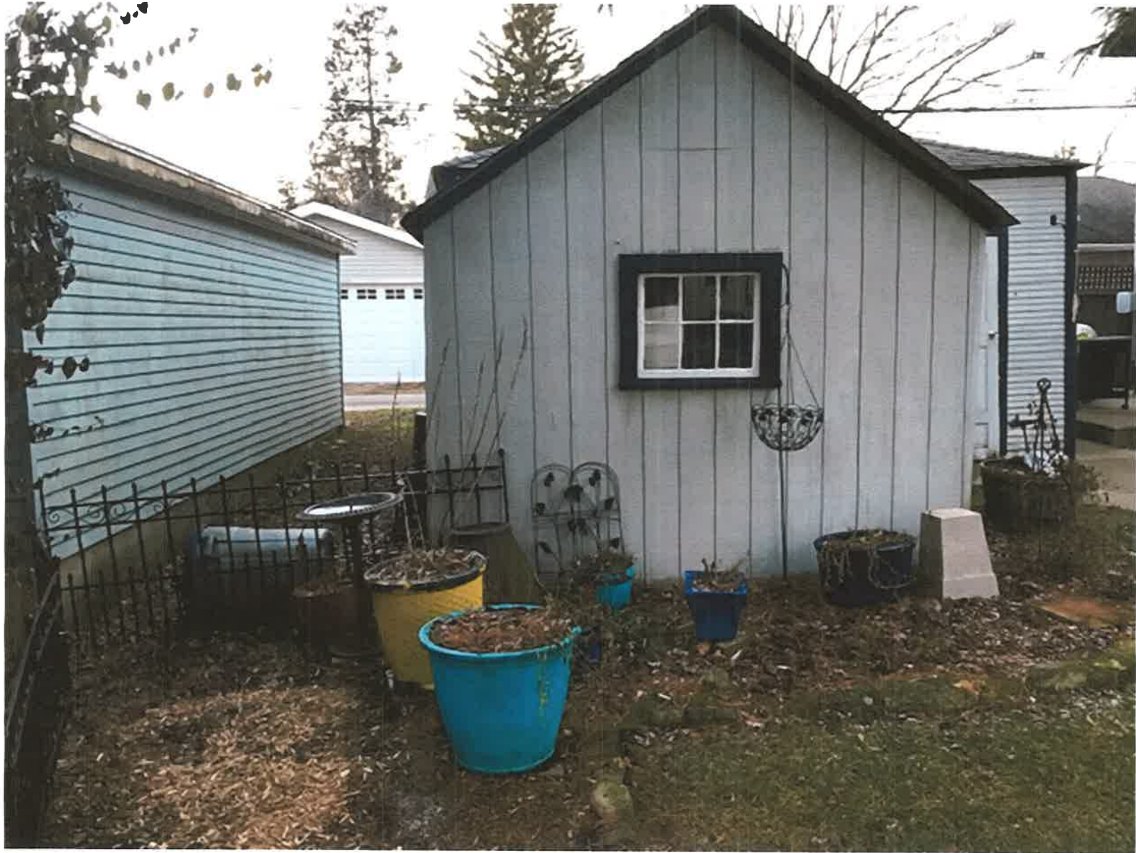
REAR OF GARAGE WITH ATTACHED SO CALLED SHED FACING EAST SHOWING SOUTH SIDE AND NORTH SIDE
