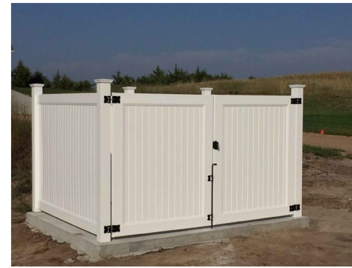
6' HIGH VINYL FENCE TRASH ENCLOSURE
