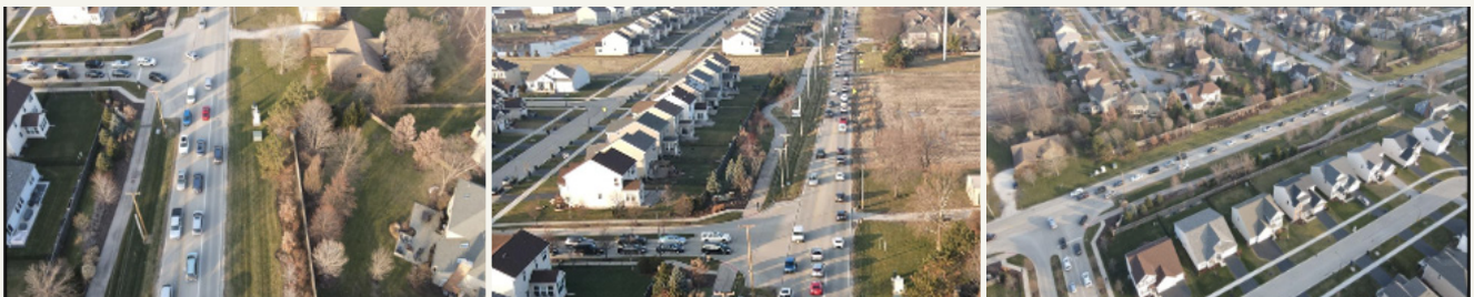
Figure 4: These photos illustrate the traffic congestion caused by just 200 vehicles moving north and southbound on 248th Ave. For comparison, ICN's Phase 1 Friday services add 1,280 vehicle trips in 2 hours with 640 arrivals and departures expected in a 15-minute timeframe.
