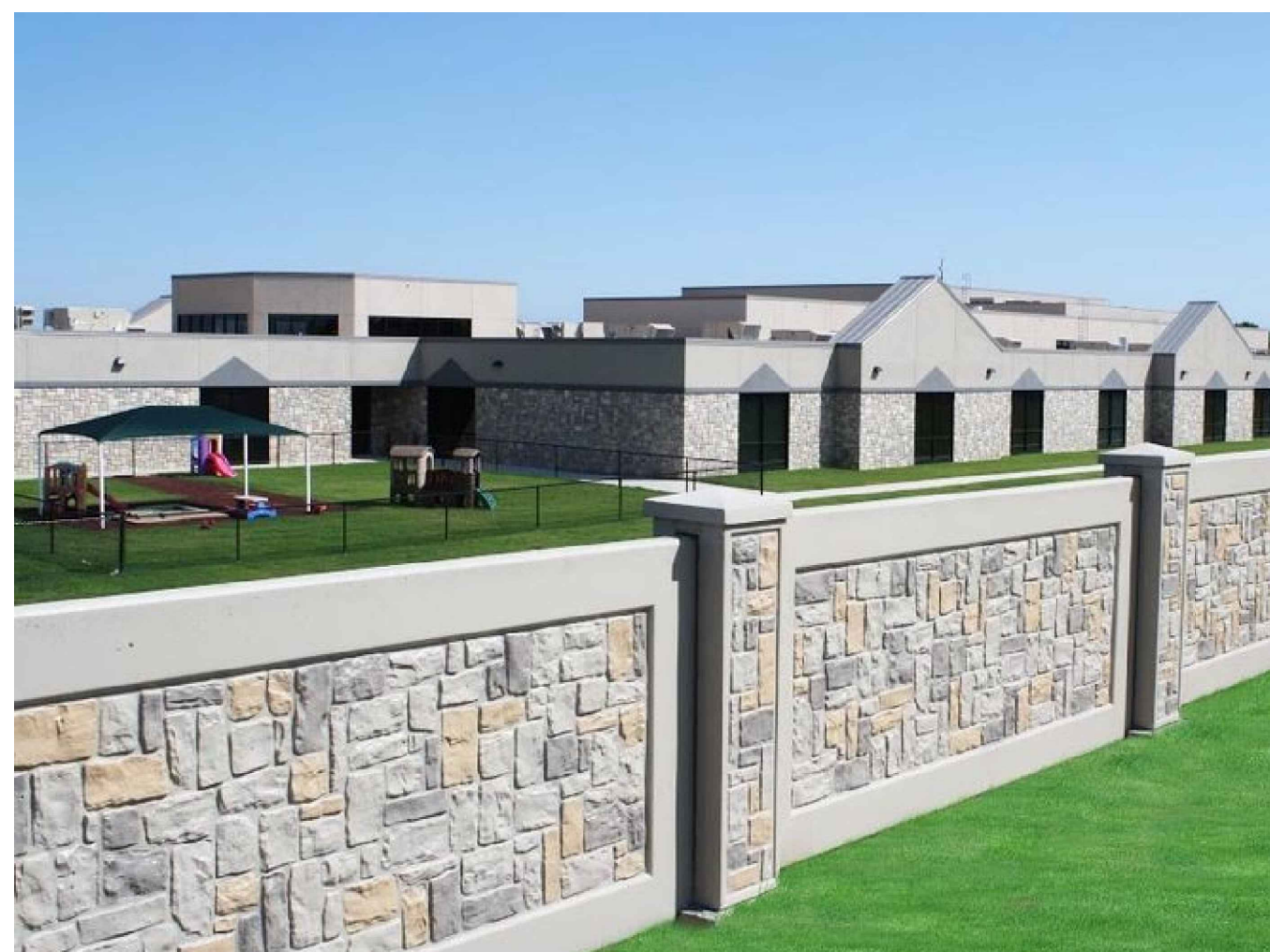
PRE-CAST CONCRETE SCREEN FENCE
