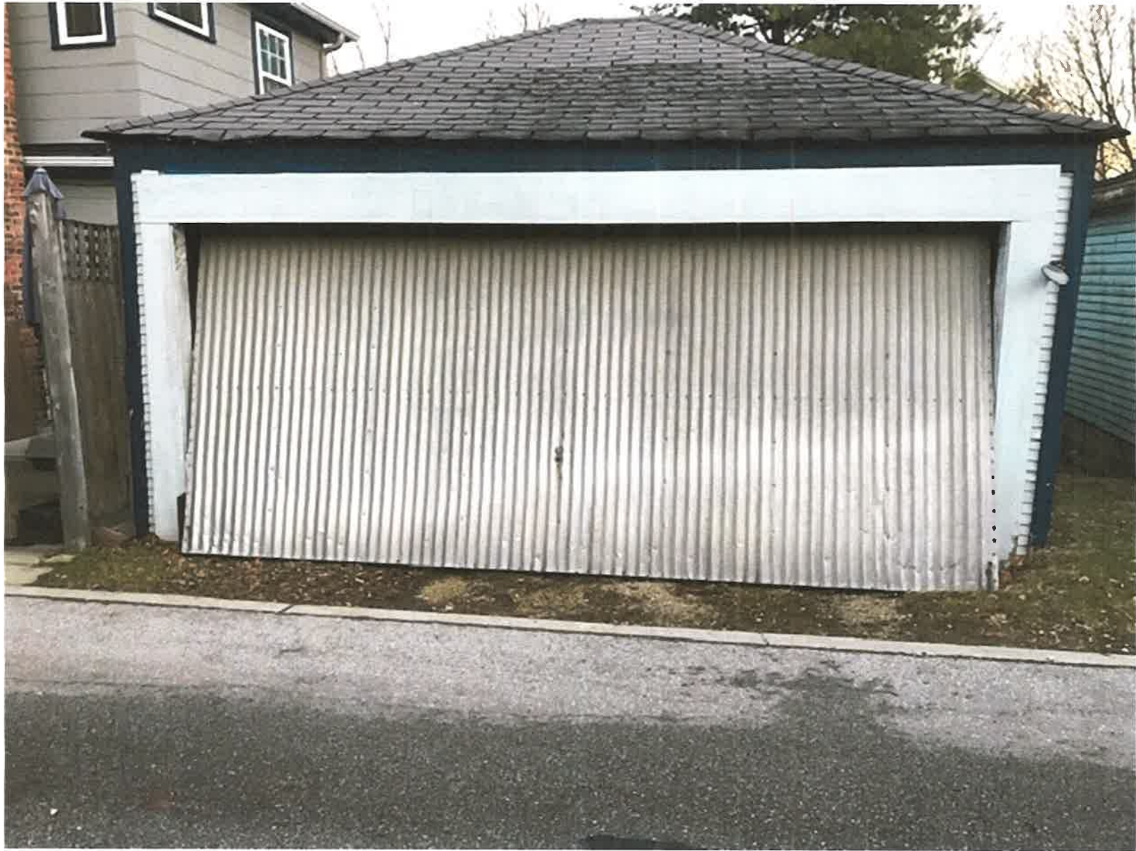
ALLEY ENTRANCE TO GARAGE FACING WEST
