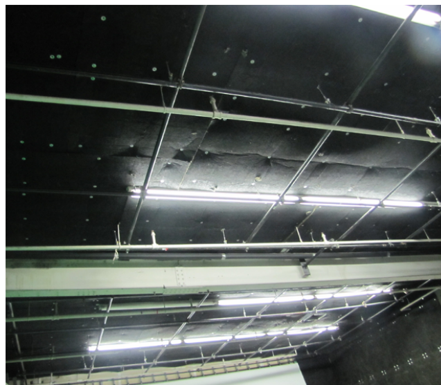
Typical installation of Owens Corning SoundSelect board (without dome caps over insulation pins)
