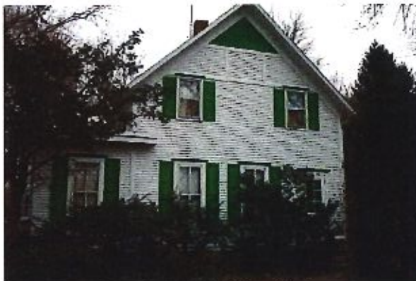
Existing Farm-Style Home proposed to be demolished
