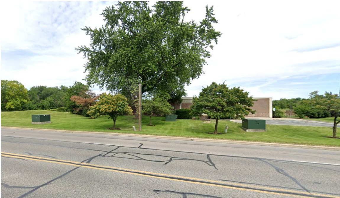
Figure 1. Looking at the west building wall from Washington Street
