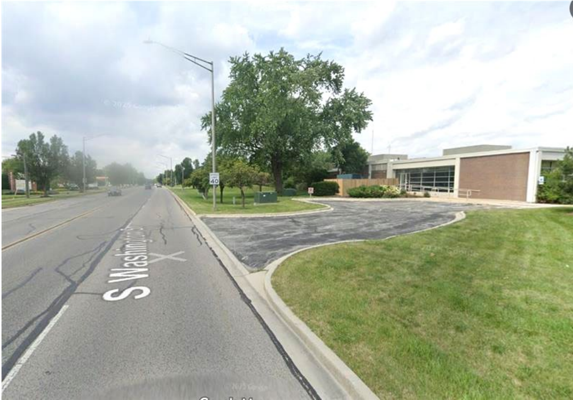
Figure 2. Looking at the west building wall from Washington Street with New Fence and Generator
