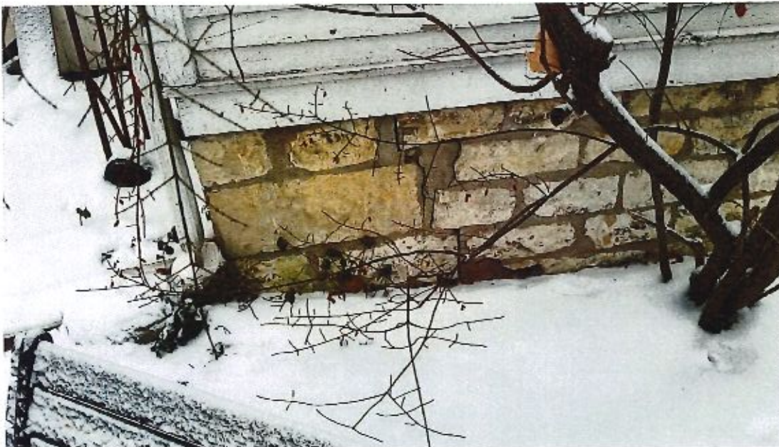
Image 20 – Stone foundation with signs of patching
