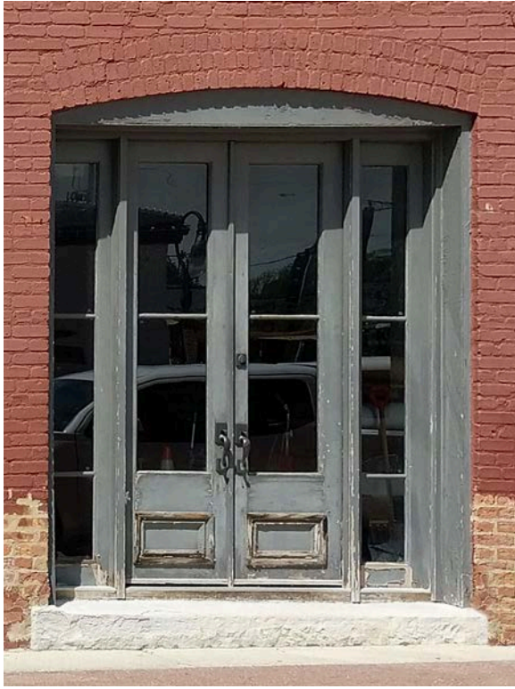
“Workshop” doors and stone step, 2024 —Naperville Preservation, Inc.
