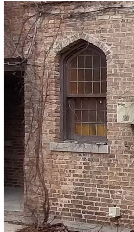
Mortuary window, 2024 —Naperville Preservation, Inc.
