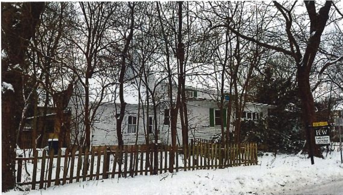
Image 3 – East addition from northeast corner
