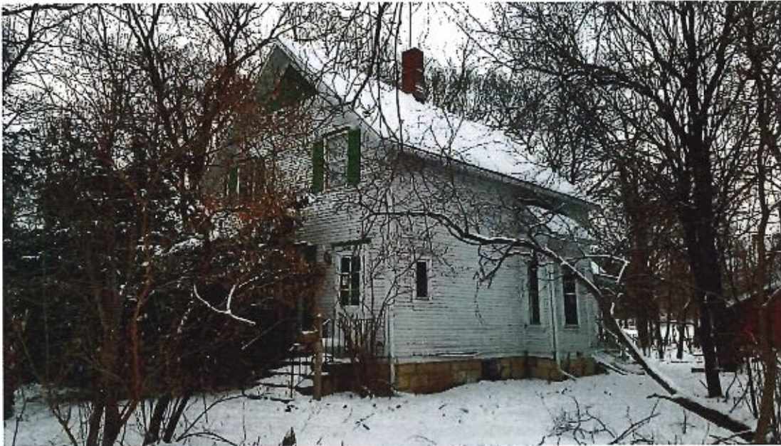
Image 1 – Existing house from southwest corner
