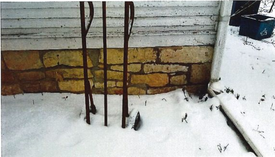
Image 19 – Stone foundation with signs of patching
