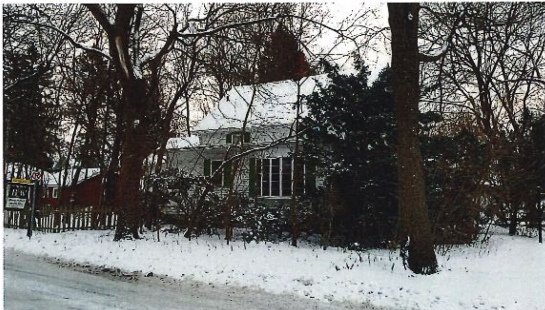
Image 2 – North addition from northwest corner
