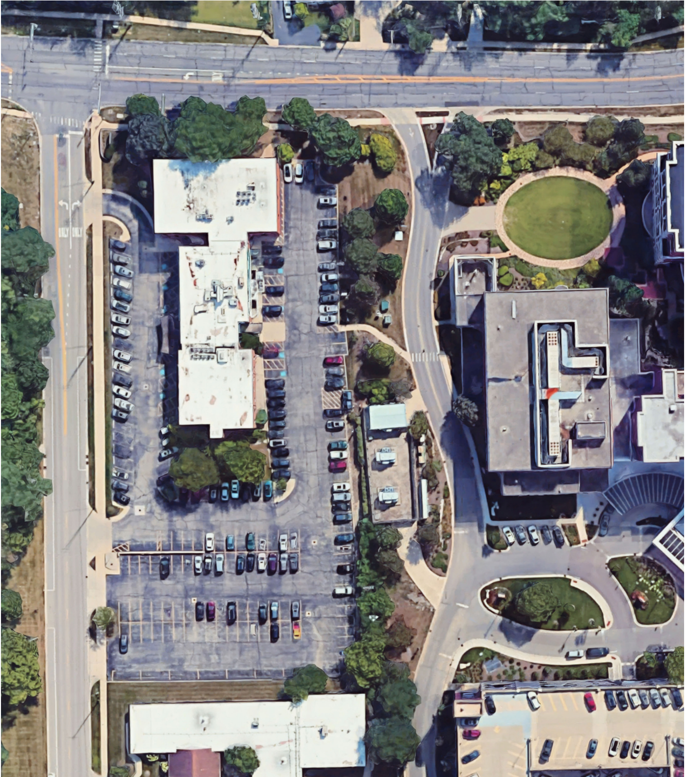
Figure 1: Current Aerial View of 10 Martin Ave
