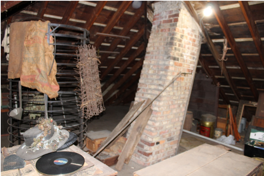
Attic, view northwest. The basement furnace vents through this brick chimney.
