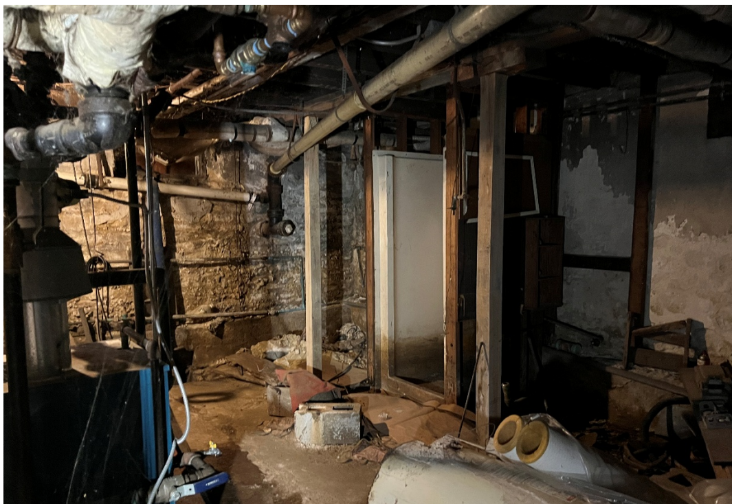
Views of the basement showing stone foundation (left) of the original 1850s house on this property.
