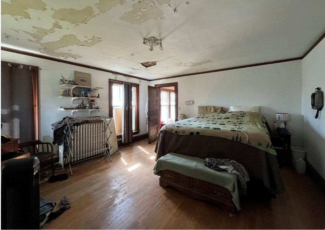
Bedroom 1, view southeast.
