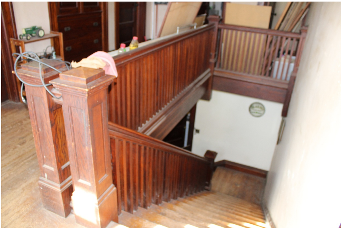
Front hall stairway at second floor level.
