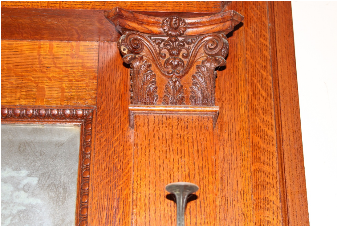
Detail of oak mirror in front stair hall showing egg and dart molding and Corinthian pilaster.
