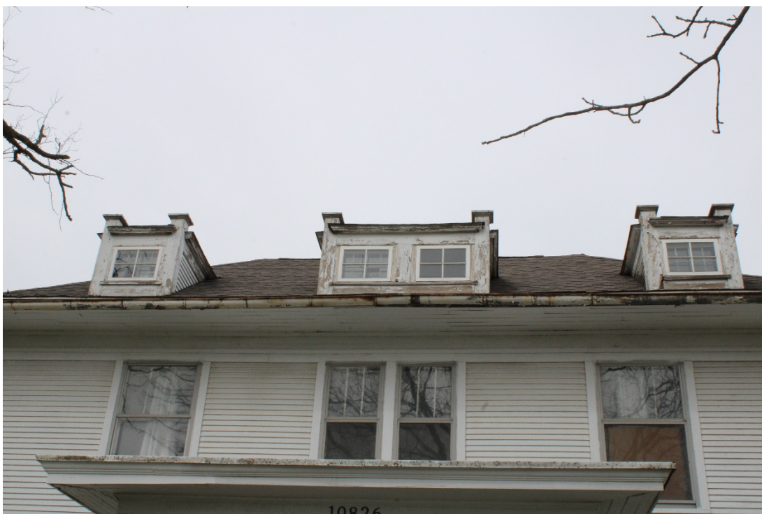
Three-over-one windows and dormers on the front facade.
