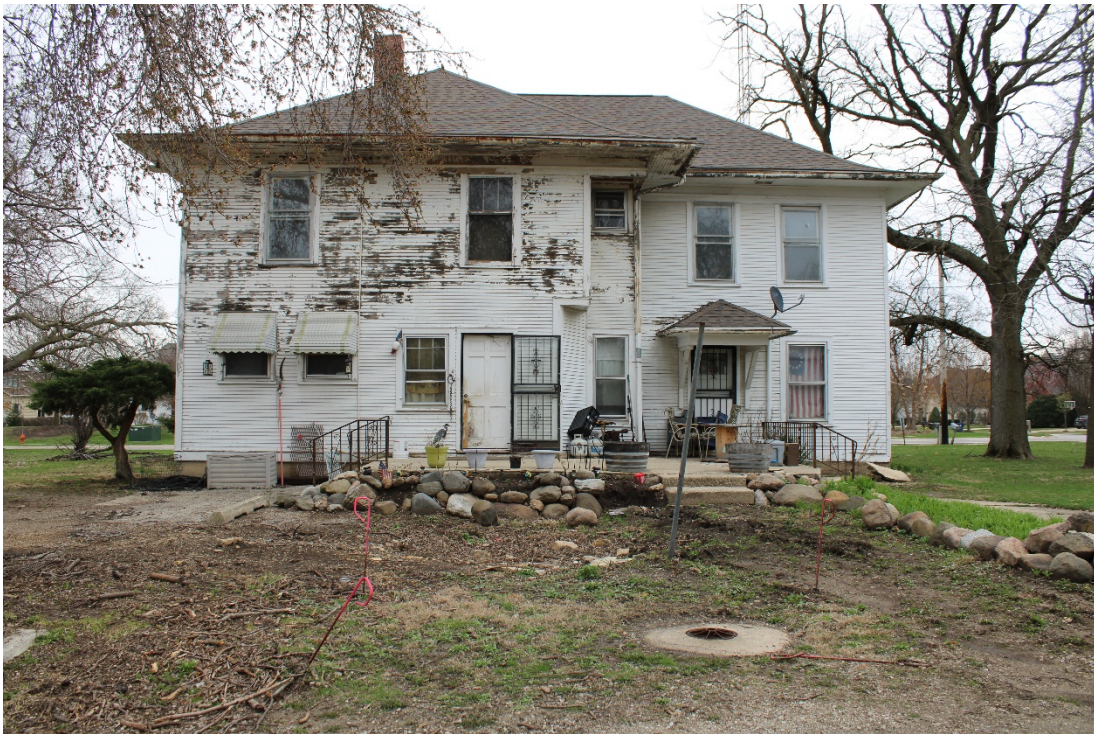
Rear (west) façade, view east.
