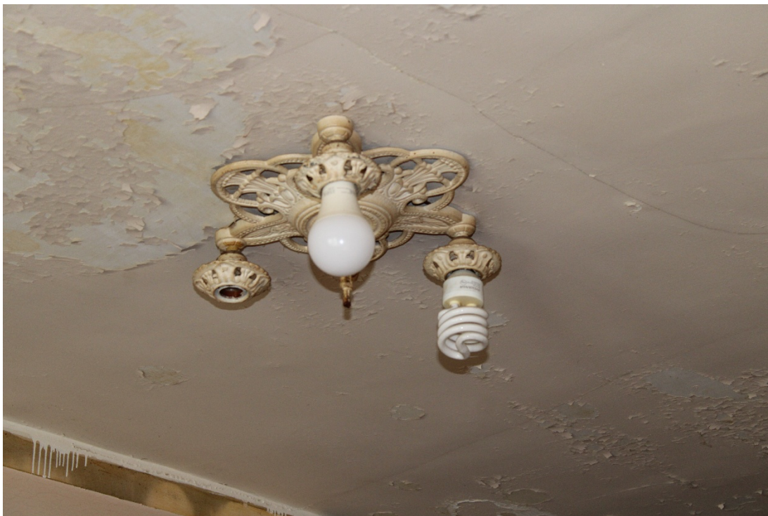
Ceiling light sconce in second floor stair hall.
