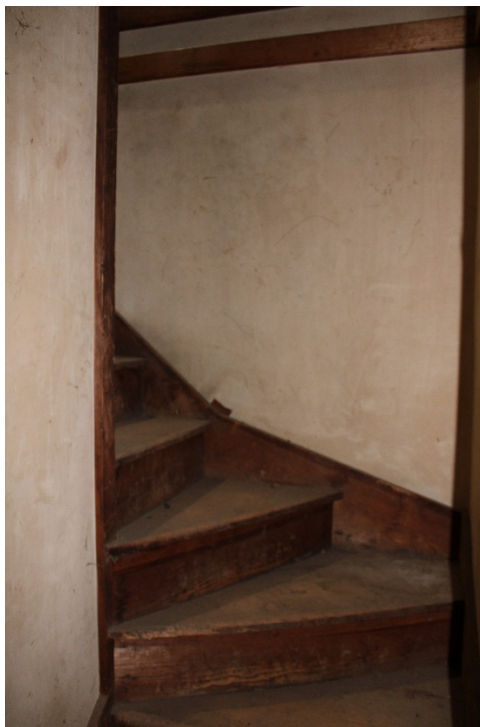
Stairway to attic.
