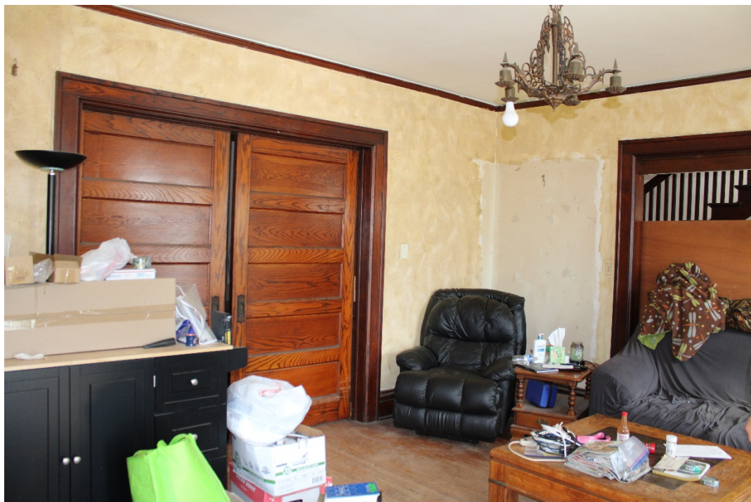
Front parlor showing original wood paneled pocket doors, view northwest.
