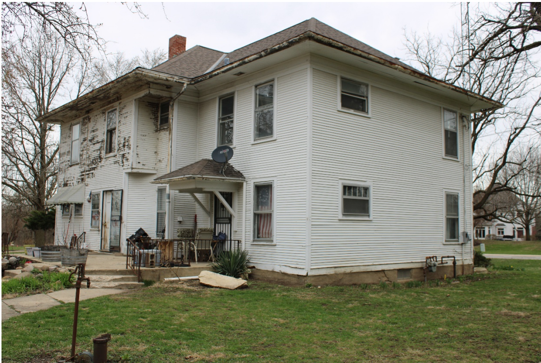
Rear (west) façade and south façade, view northeast.
