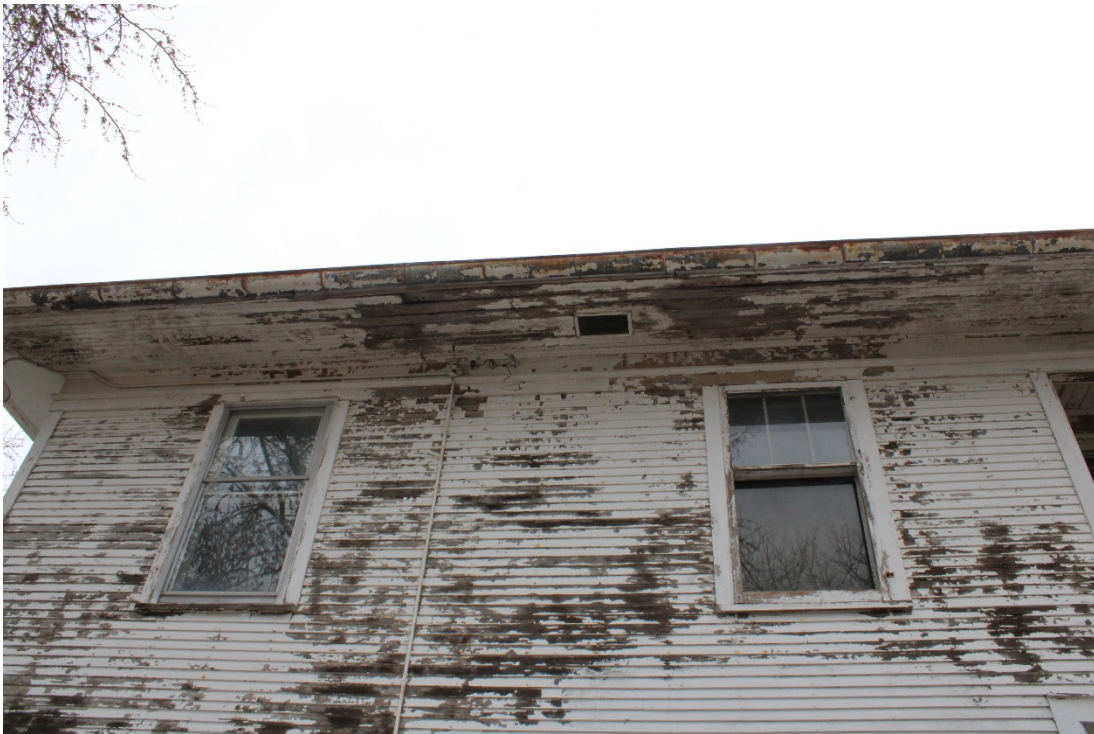
Detail of wood clapboard and windows.
