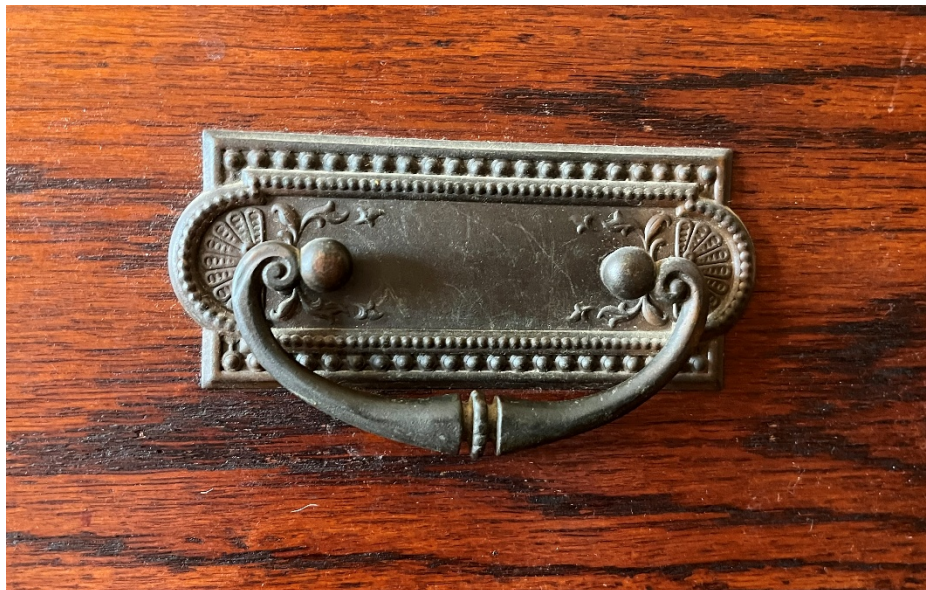
Drawer pull on second floor linen cabinet.
