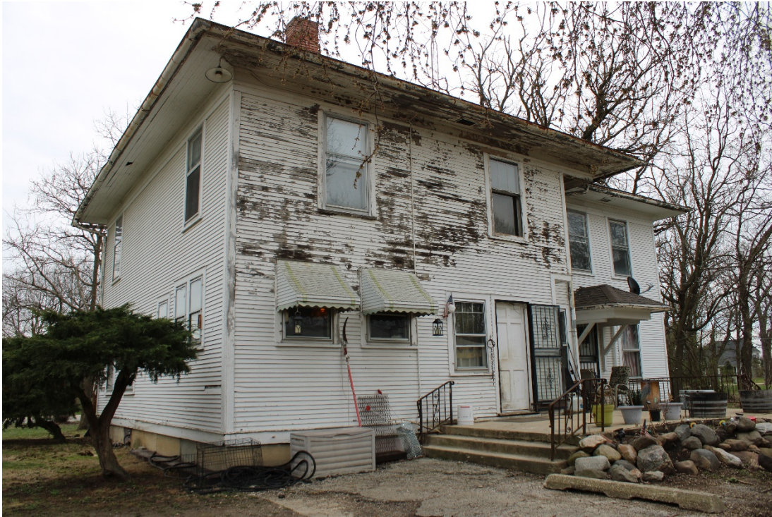
North (left) and rear facades, view southeast.
