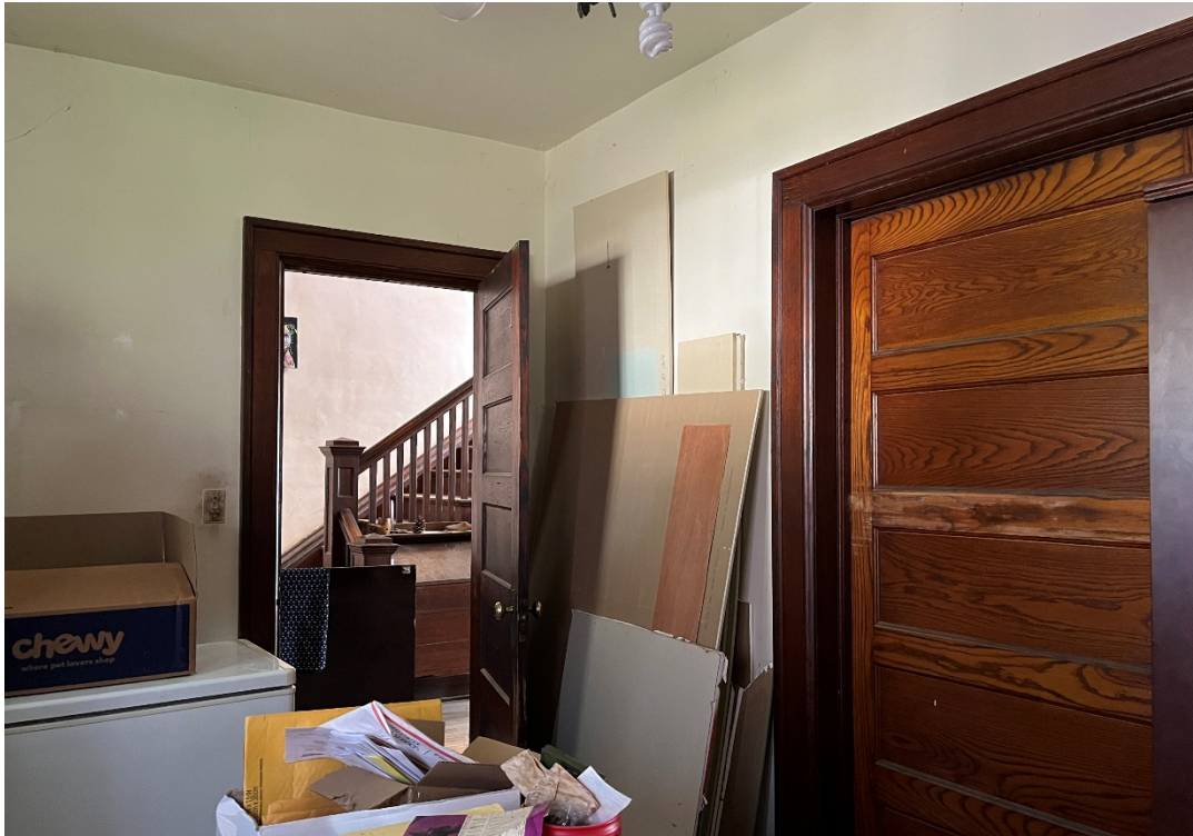
Rear parlor showing a portion of the pocket doors on the right, view north.
