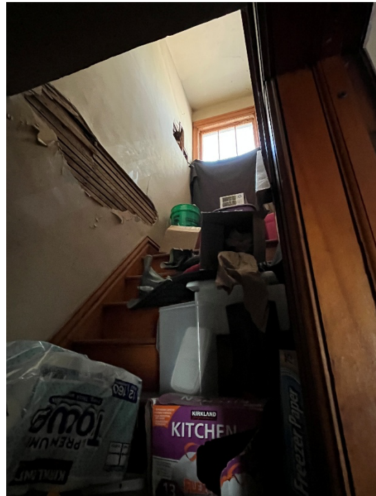
Rear stairwell to second floor.
