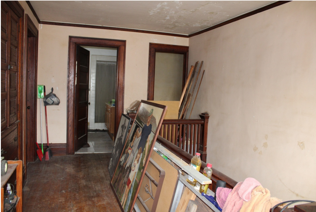
Second floor stair hall, view west toward doors to bathroom (left) and rear stair landing.
