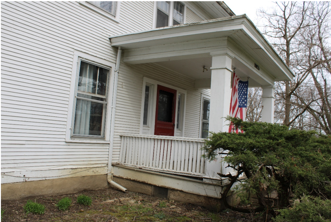
Front façade porch, view northwest.
