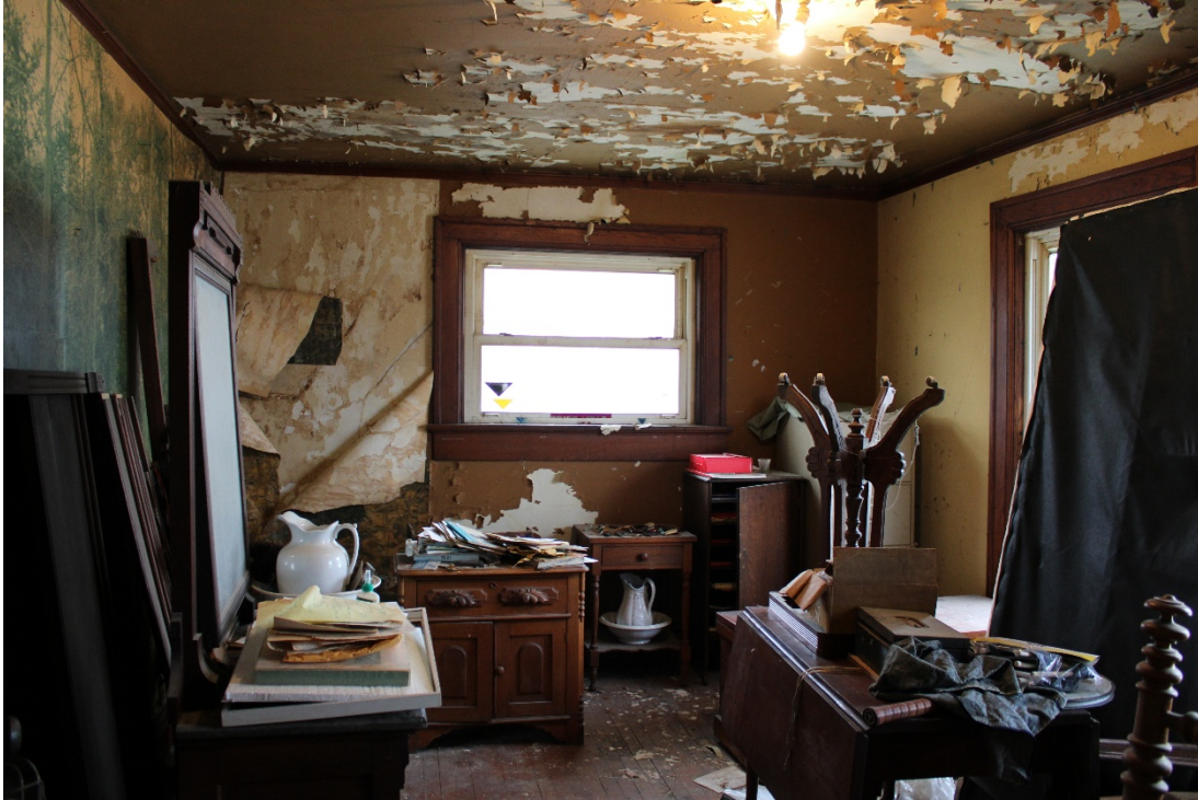
Bedroom 3, view south.
