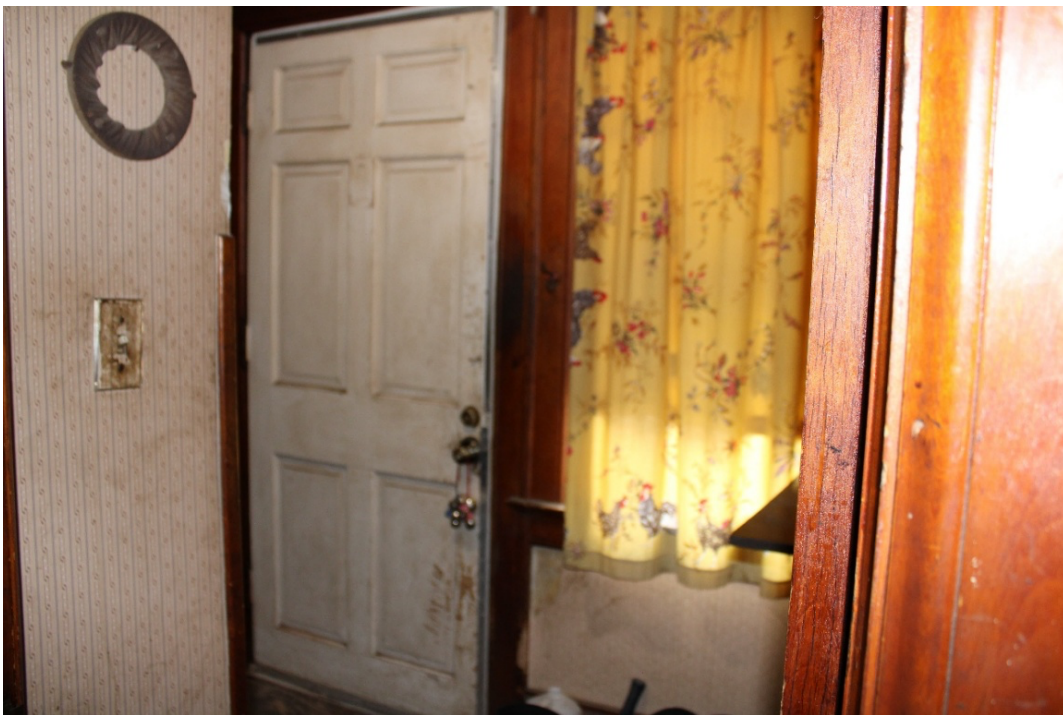
Rear vestibule, view southwest.
