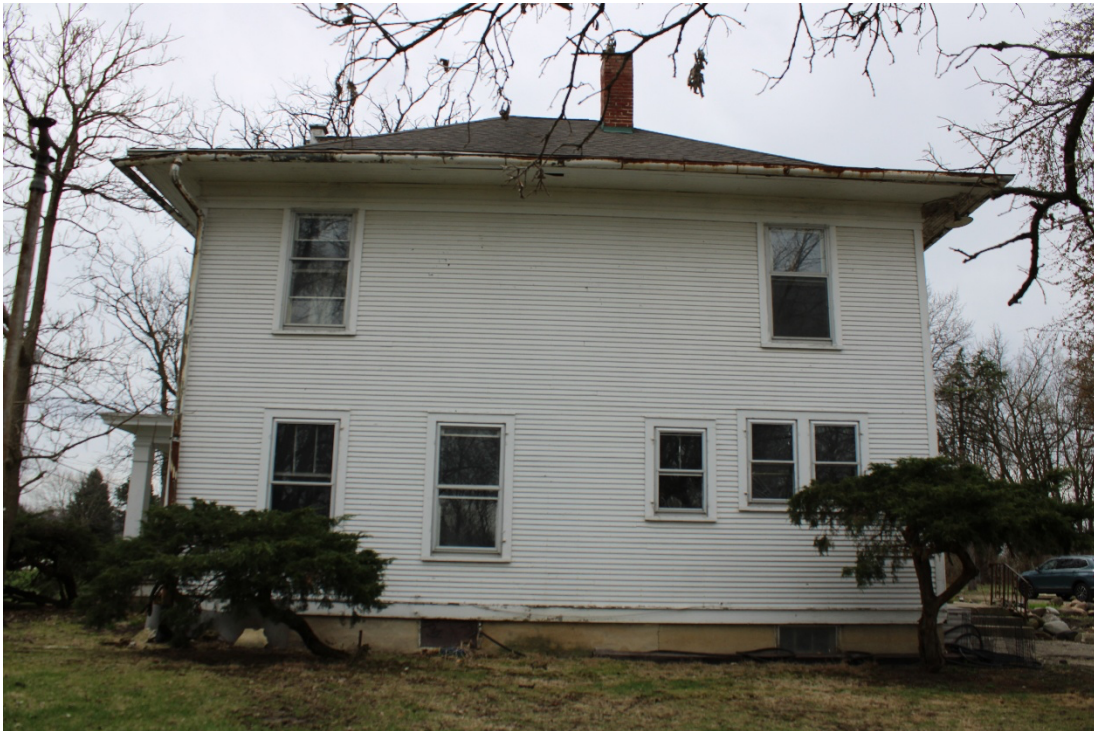
North façade, view south.
