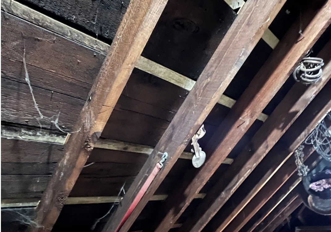
Detail of attic rafters.
