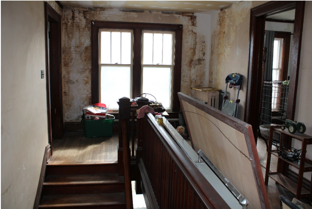
Second floor stair hall, view east.
