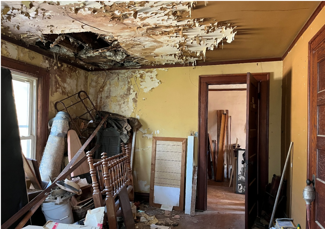
Bedroom 3, view north.
