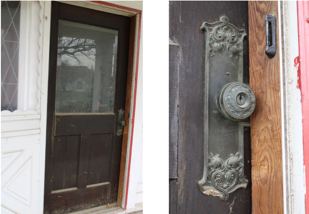
Front door and detail of its doorknob.
