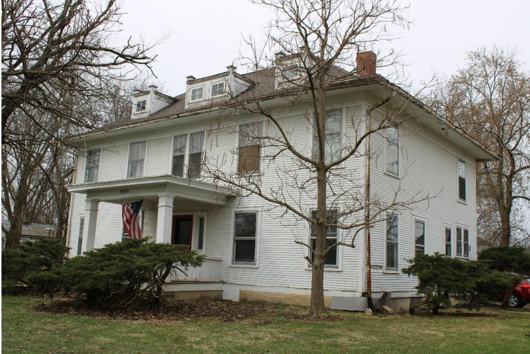
Front (east) and north facades, view southwest.
