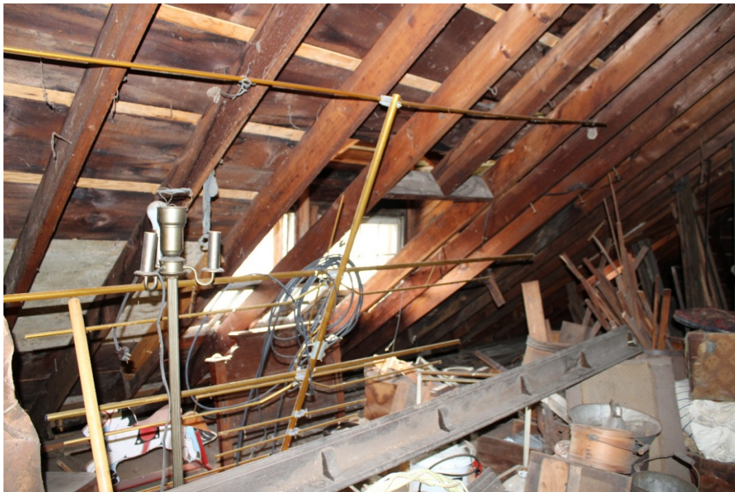
Attic, view southeast.
