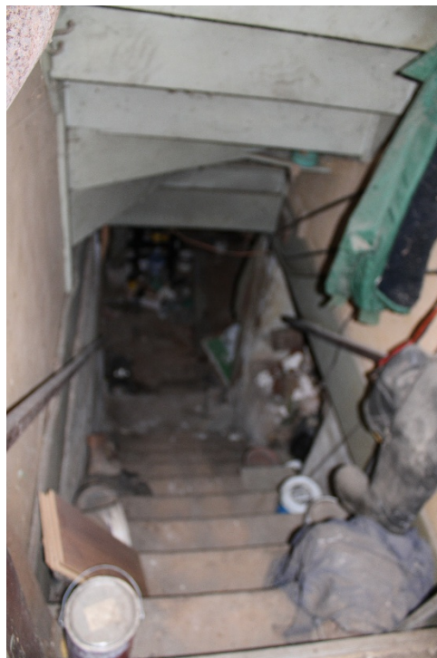
Stairway to basement.
