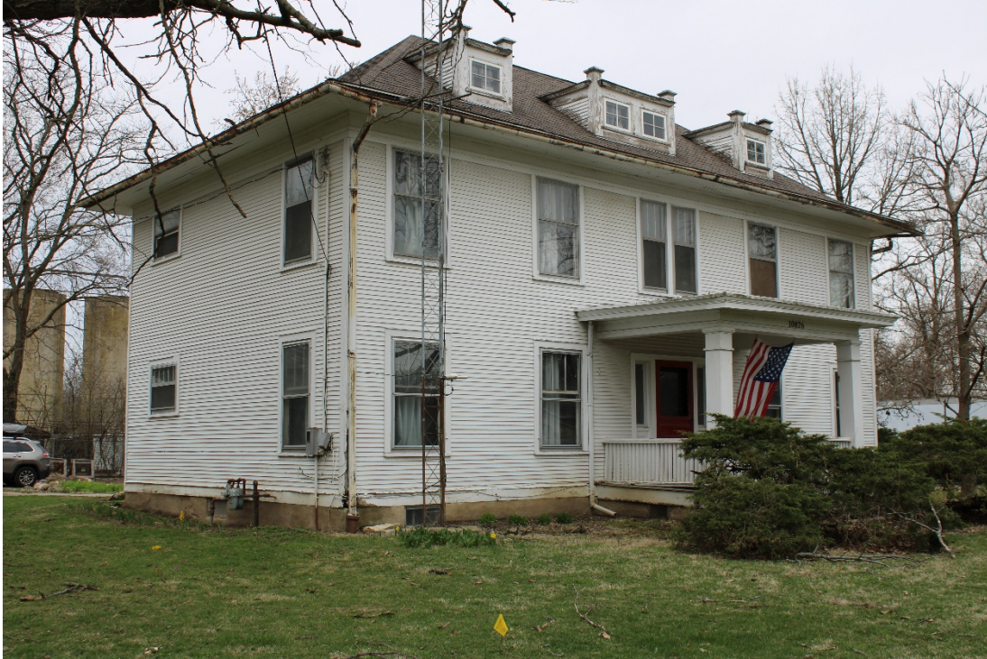
South (left) and front facades, view northwest.
