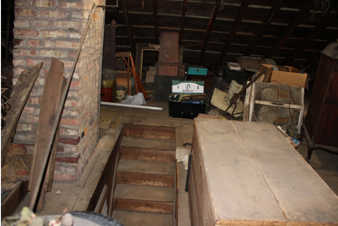
Attic, view north.
