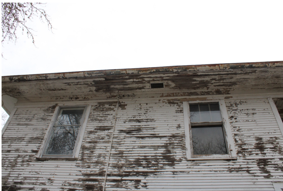
Detail of wood clapboard and windows.
