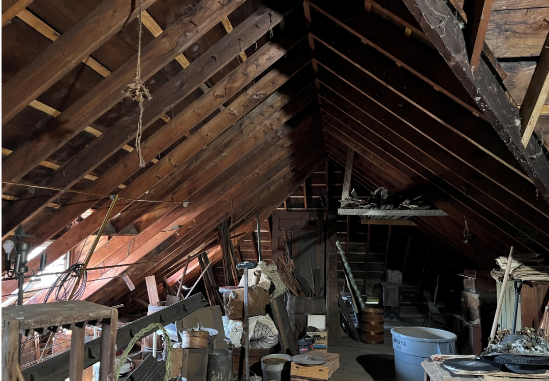
Attic, view south.
