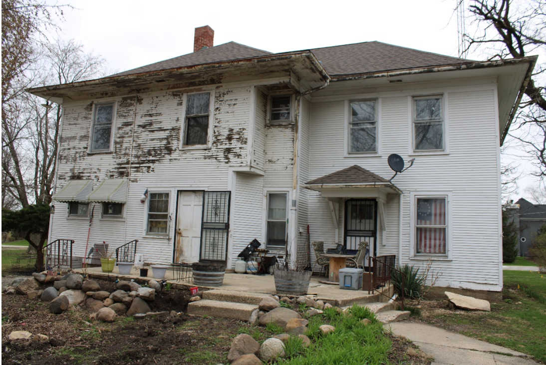
Rear (west) façade, view northeast.
