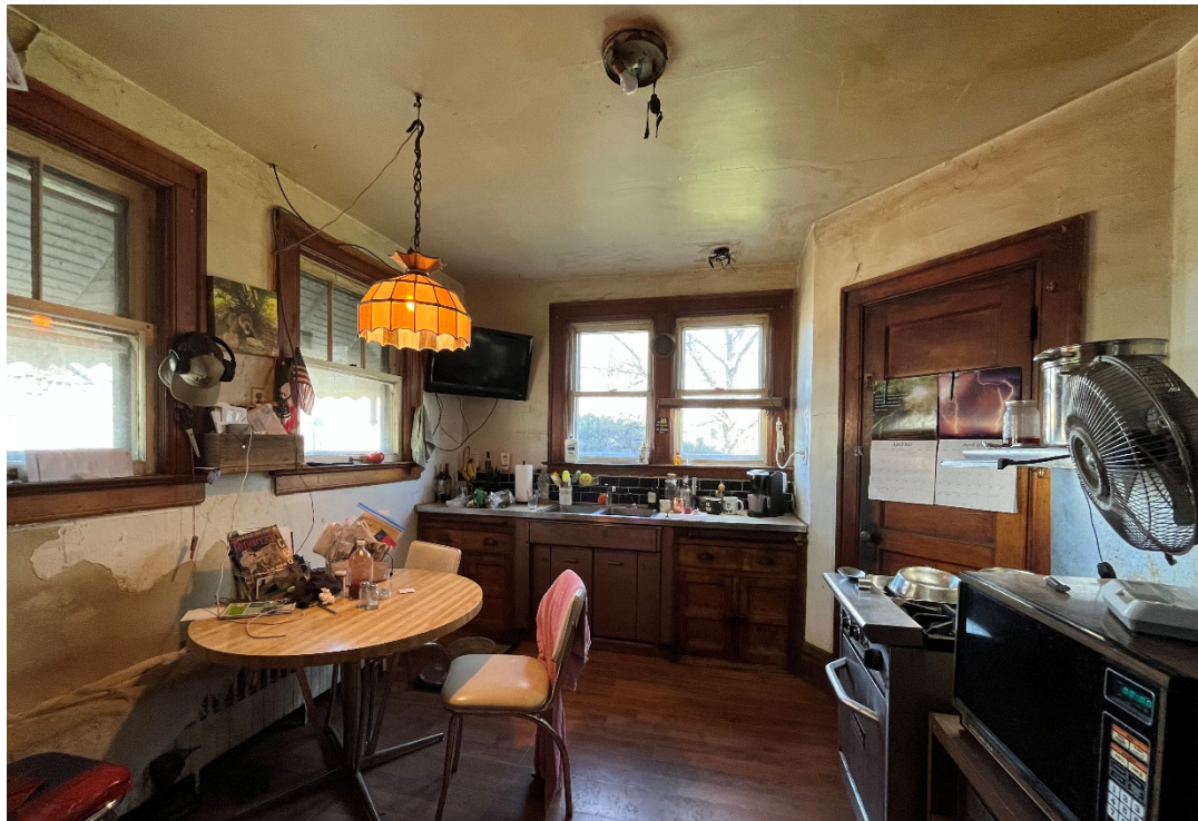
Kitchen, view north.
