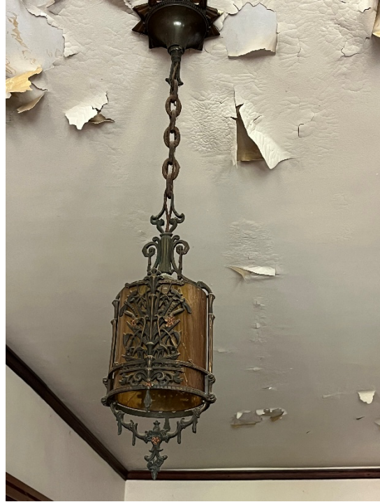
Ceiling light fixture in front stair hall.
