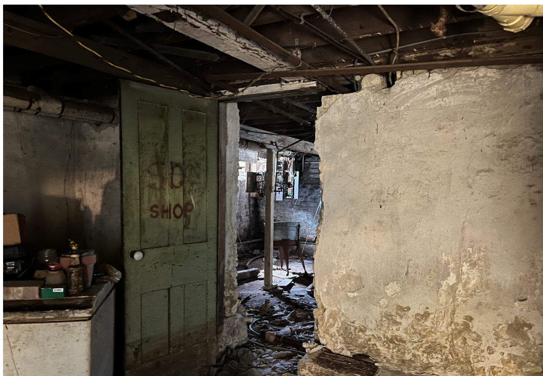
Views of the basement showing stone foundation (left) of the original 1850s house on this property.
