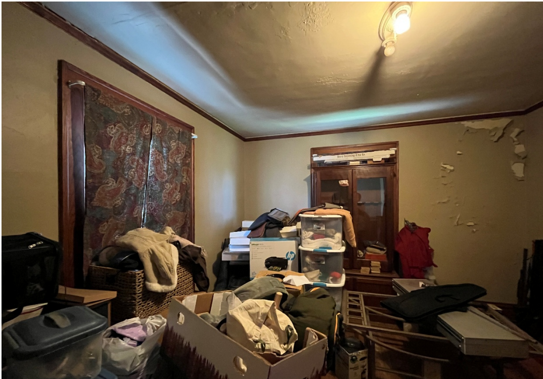
Bedroom 4, view north.
