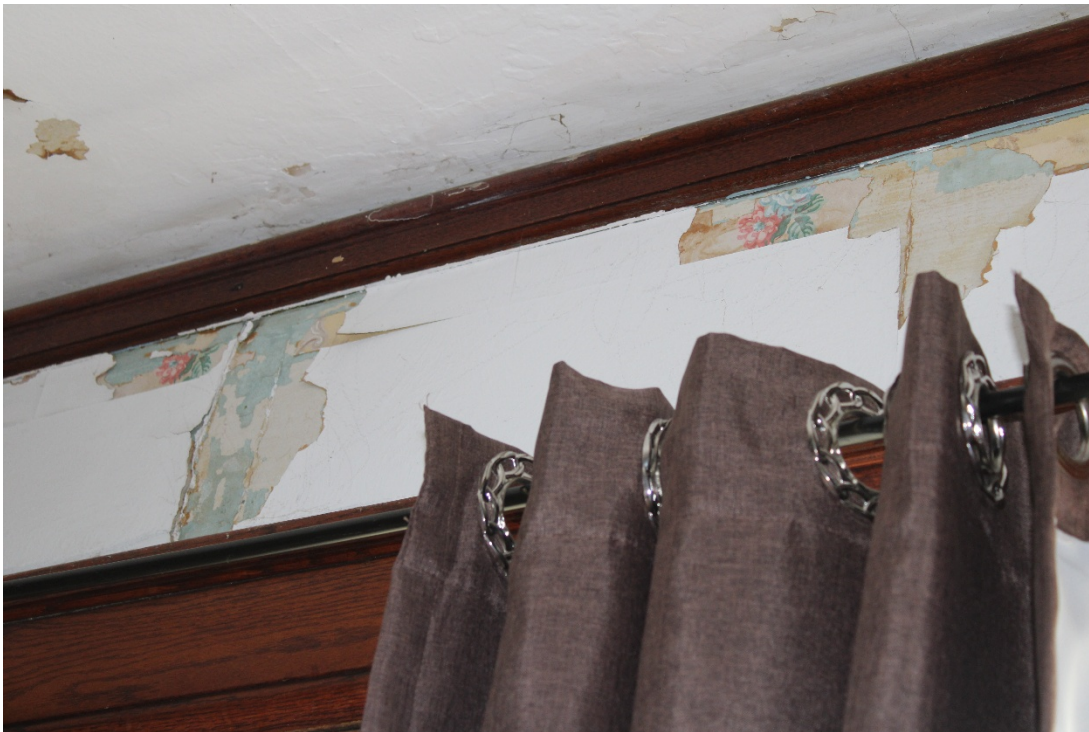
Detail of bedroom 1 plaster wall showing original wallpaper beneath the paint.
